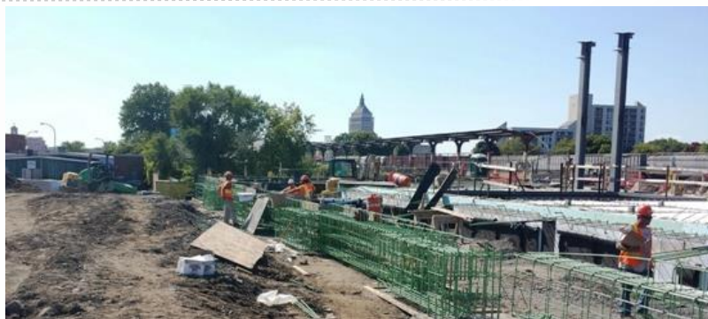
Rochester station under construction in September 2016 (Photo: NYSDOT)
