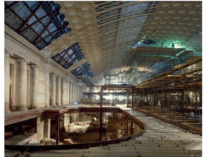
1910 photo of concourse (top), 1980s photo of alterations to concourse floor, Source: Library of Congress
