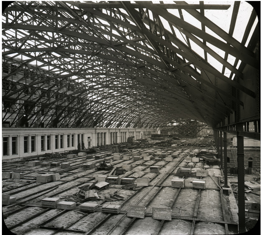
Construction of original concourse floor, Source: Historical Society of Washington, DC
