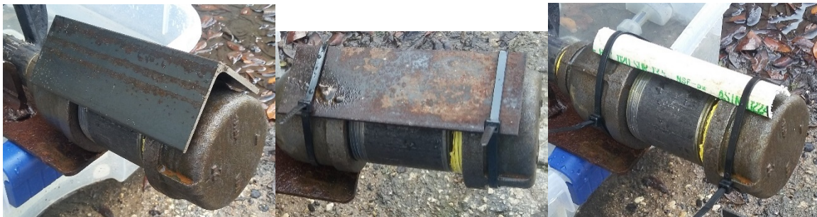
Figure 17. Select Covering Methods to Reduce Spray; 2-in. Angle Iron, 2-in. Wide Plate, 1-in. Diameter PVC Tubing Split Lengthwise
