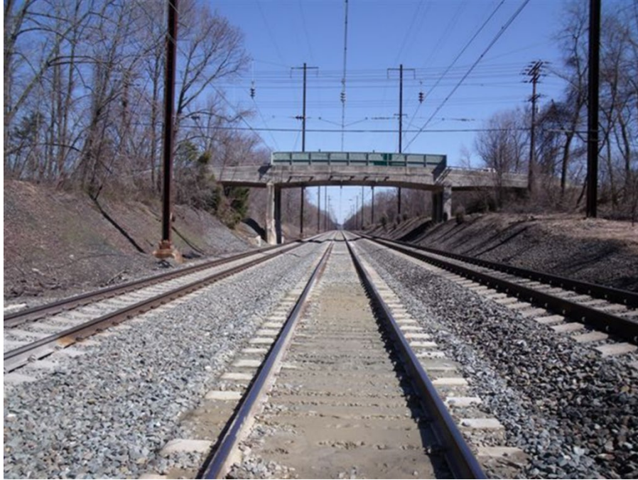
Figure 1: Amtrak Oakington Road site MP 62.6 to 61
