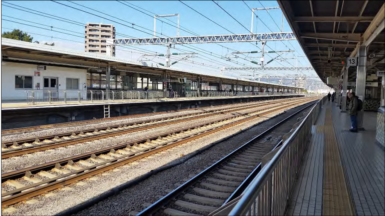
Figure 2-12: Japanese Station Platform Infrastructure
