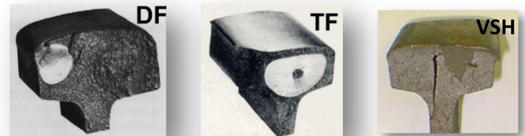
Examples of Rail Flaws Relevant to Safety (Left to Right: Detail Fracture, Transverse Fissure, and Vertical Split Head)
