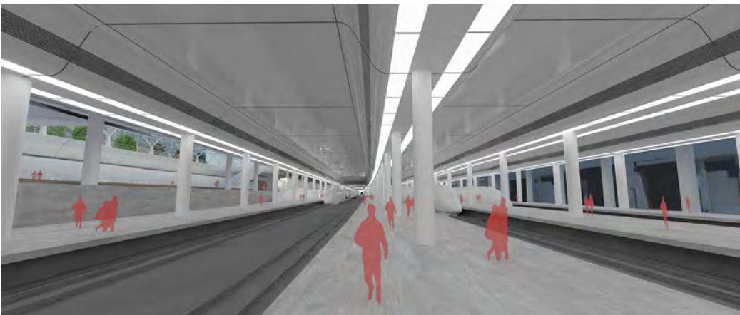
Figure 71. View from run-through platform with deck level at 86.25' and soffit at 70.25' (27' clear at platform)
