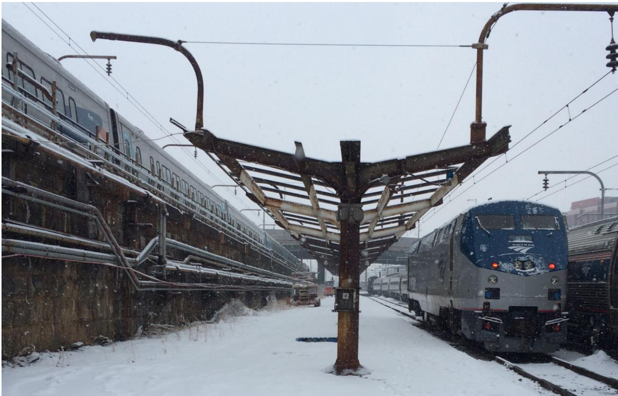
Figure 12: Track 22 locomotive pool track, and abandoned Track 21 (left)
