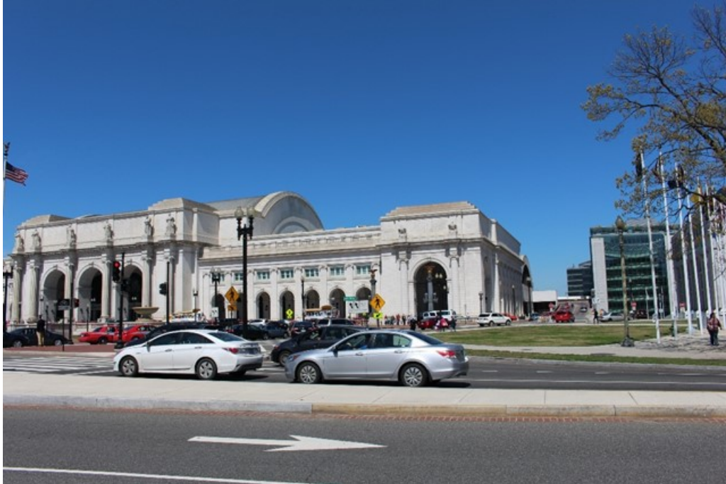
Figure 11-18. Street View Looking Northwest, towards WUS and the Project Area, from Massachusetts Avenue NE at the East Side of Union Station Plaza
