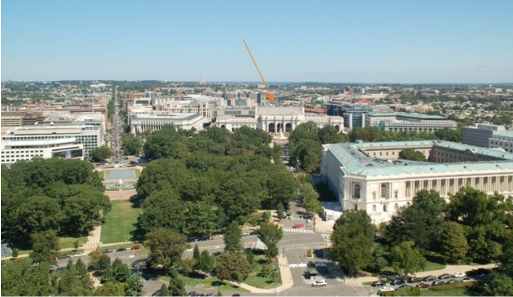
Figure 11-19. View north of WUS and the Project Area from the Dome of the U.S. Capitol Building
