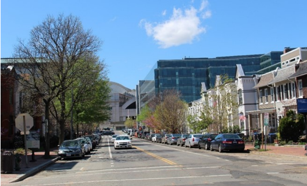
Figure 11-6. View looking west to the Project area and WUS from F Street NE and Third Street NE
