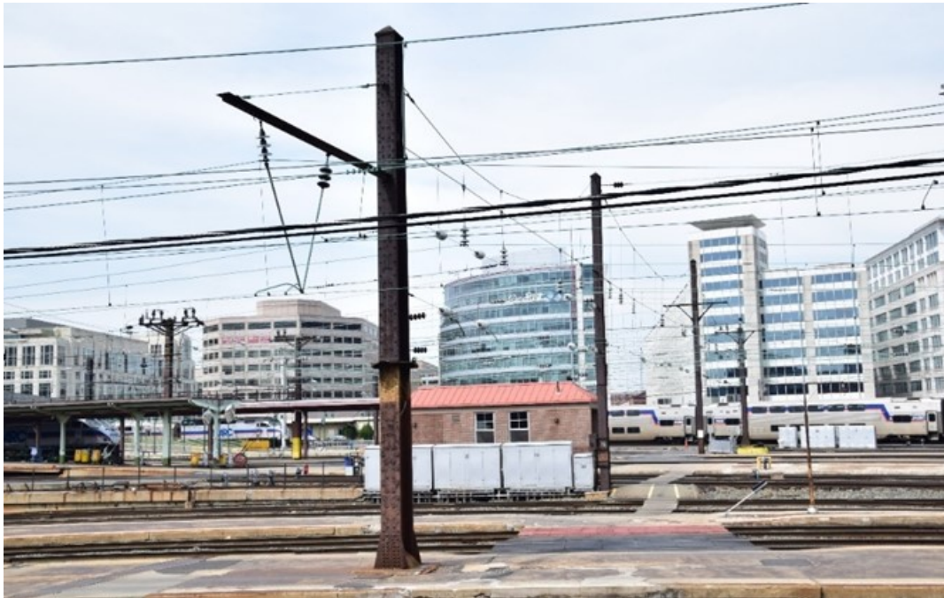
Figure 11-5. View Looking West of The WUS Terminal Rail Yard
