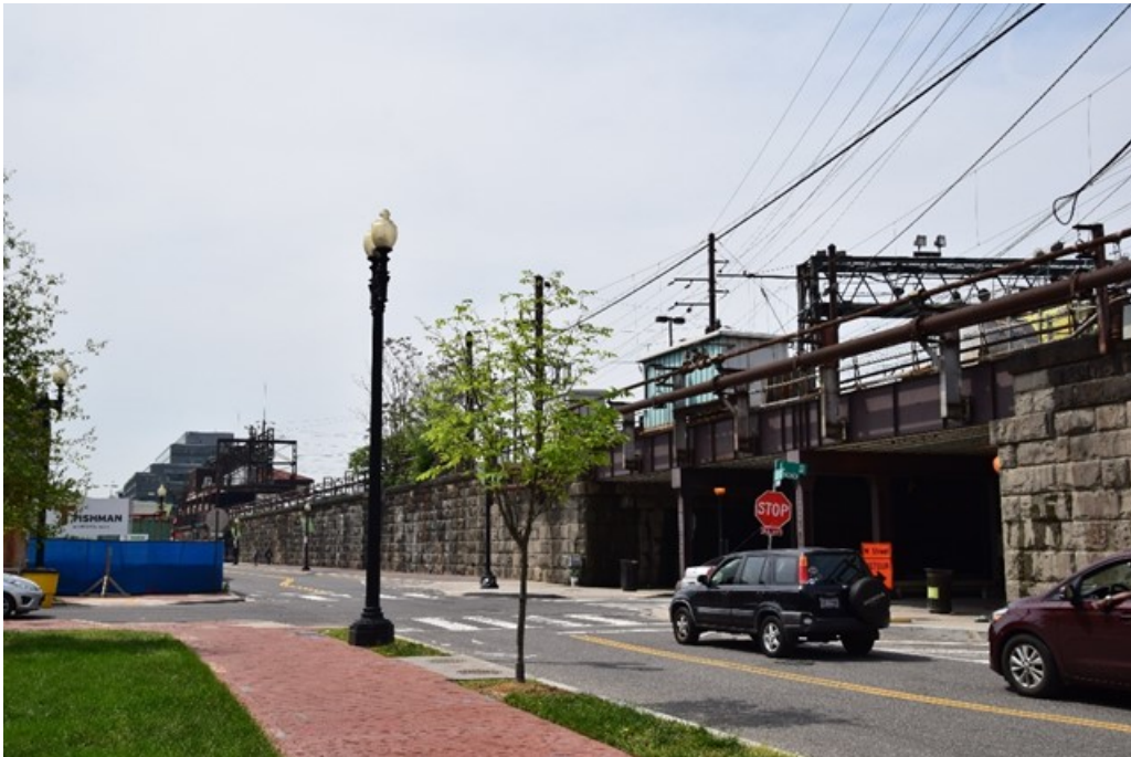
Figure 11-17. Street View Looking South, towards the Project Area, along Second Street NE from L Street NE
