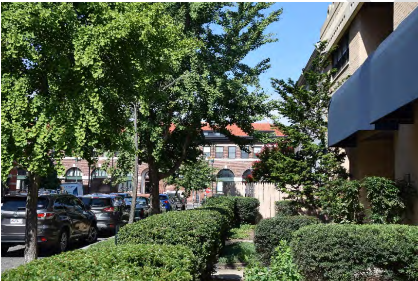
View from the south elevation of the property looking west towards the REA Building and Project Area along Eye Street NE
