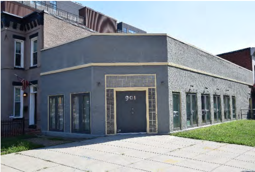
901 Second Street, view looking northeast
