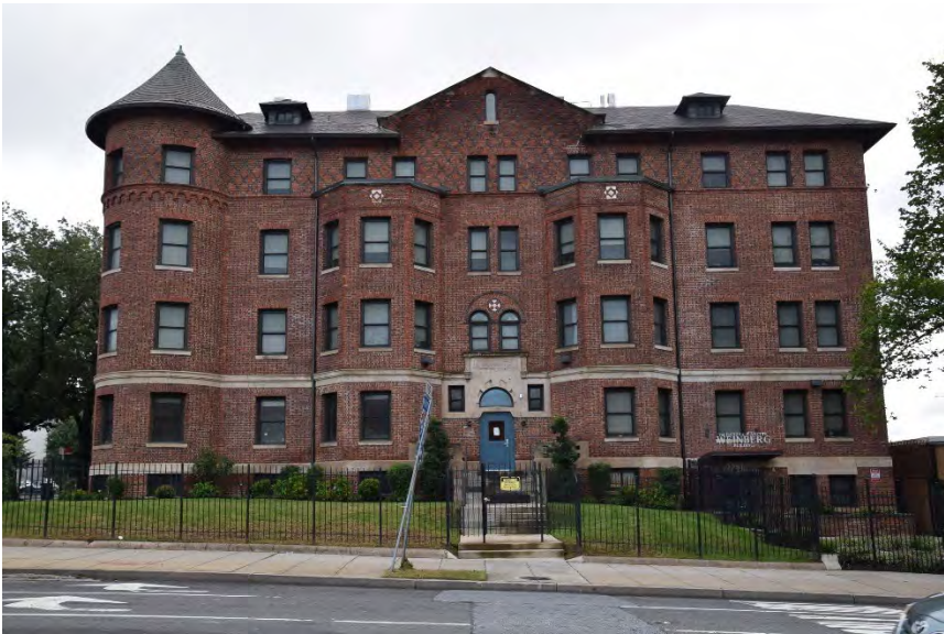
Augusta Building, view looking east
