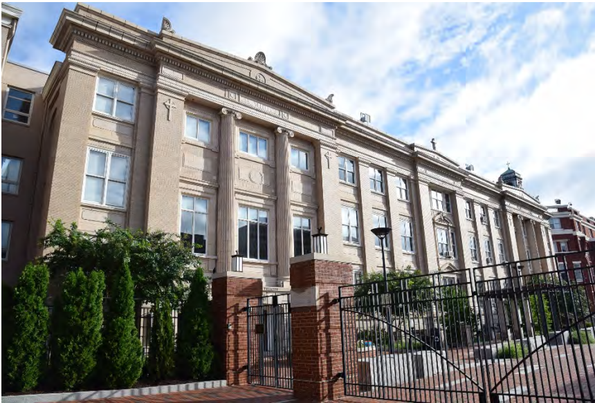
Gonzaga College High School, Dooley Hall, view looking northeast
