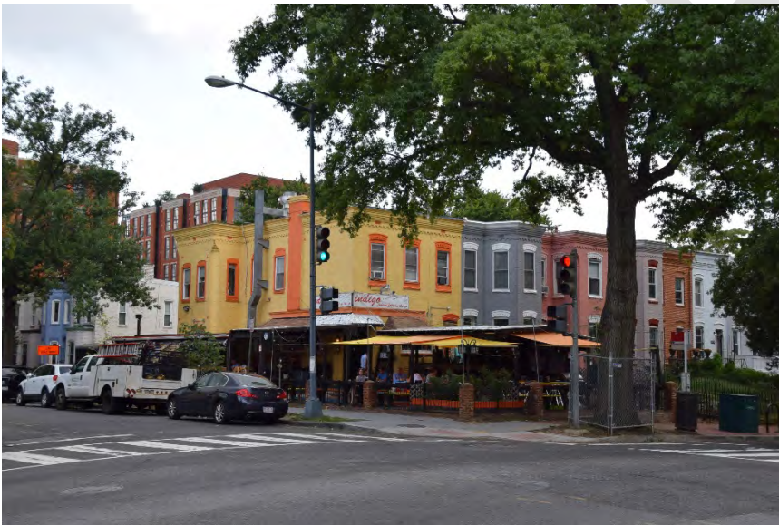
Square 750 Rowhouse Development, view looking southwest from K Street NE and Third Street NE
