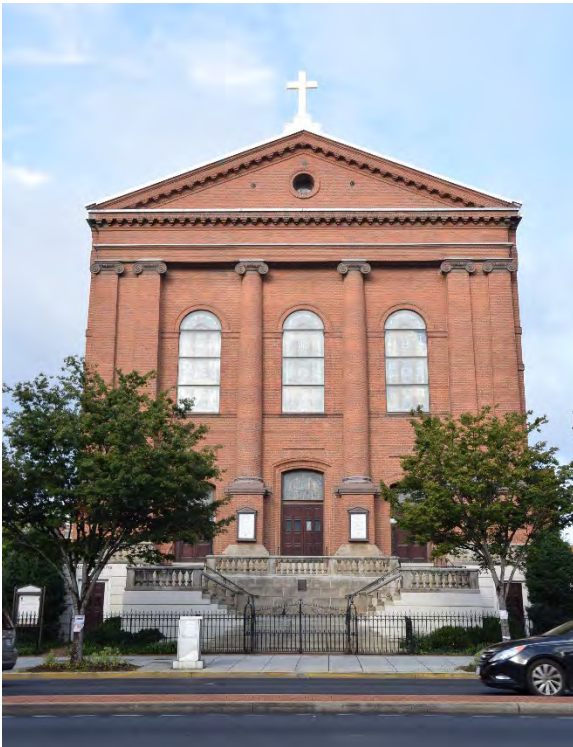
St. Aloysius Catholic Church, view looking west
