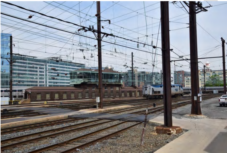
Photograph of the Terminal Rail Yard showing existing conditions of "K" Tower and several original single catenaries, looking north
