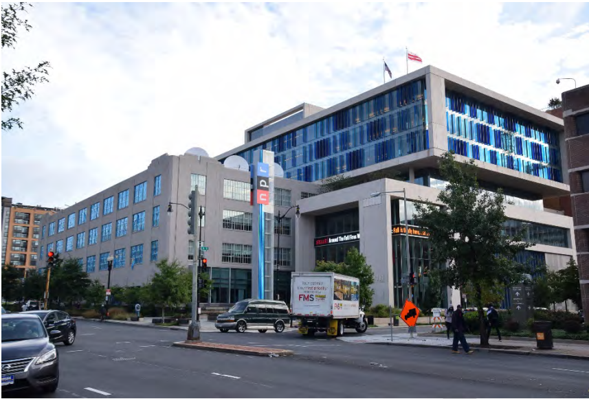
C&P Telephone Company Warehouse, view looking northeast from North Capitol and L Streets NW. The original building is on the left with an addition to the right.
