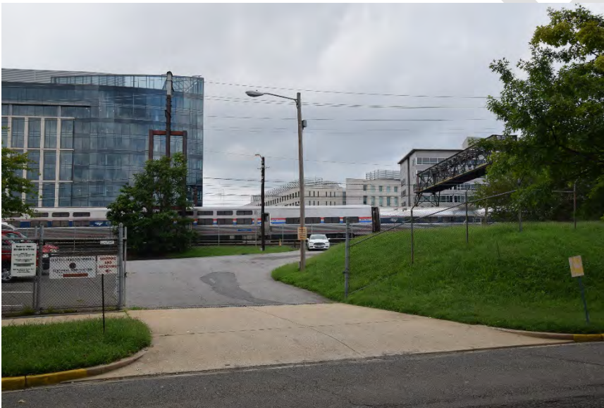
View from the west side of the building, looking west towards the Project Area. A signal bridge from the Terminal Rail Yard is visible on the right.
