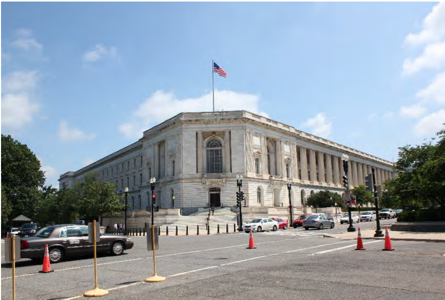
Russell Senate Office Building, view looking north
