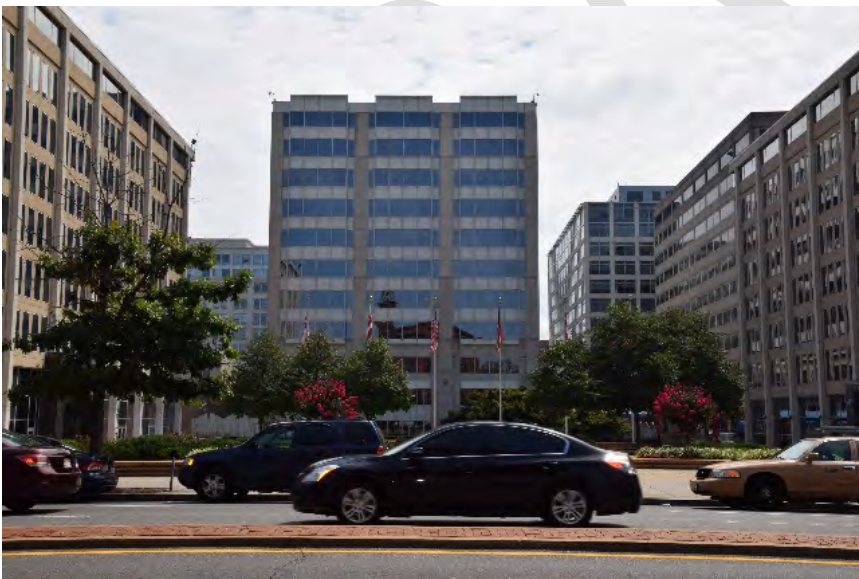
View from the east elevation of the church looking east towards the Project Area
