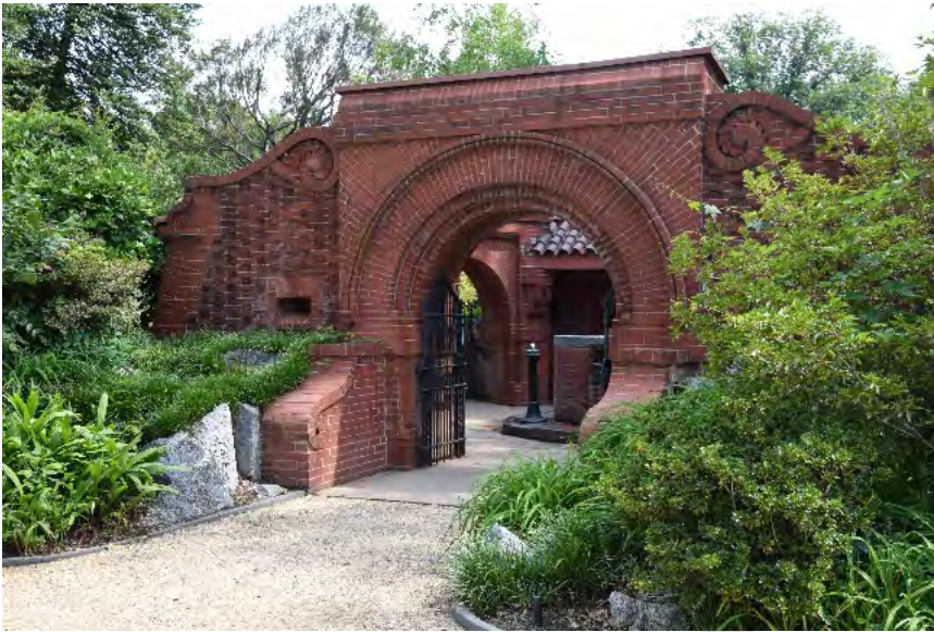
The Summerhouse located on the U.S. Capitol Grounds, view looking northeast
