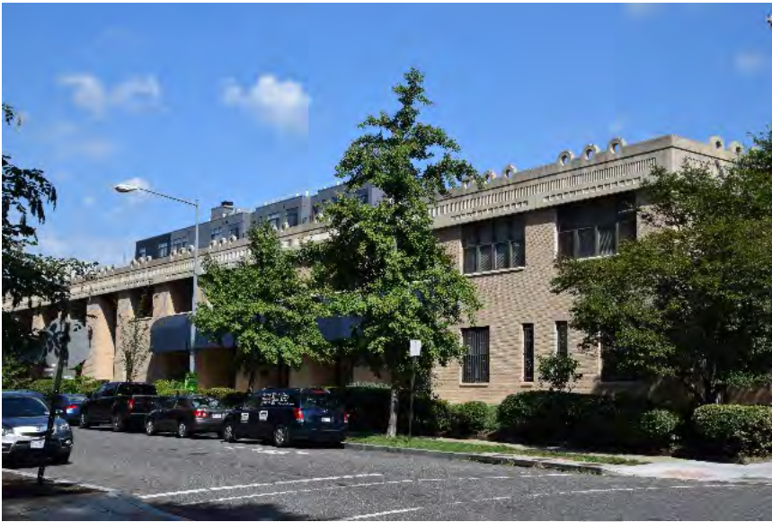
Topham's Luggage Factory (former), view looking northwest
