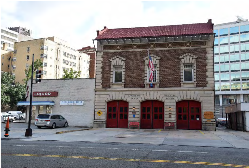
Engine Company No. 3 west elevation, view looking east from New Jersey Avenue. This property does not have a view towards the Project Area.
