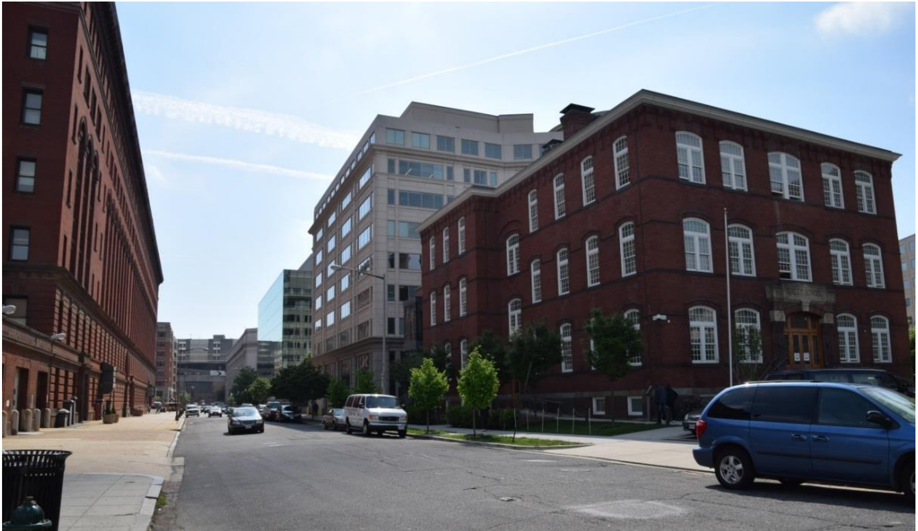
Image I. View looking east towards Union Station garage from G Street NW and Massachusetts Avenue NW with the Gales School (DC Inventory of Historic Sites) in foreground.
