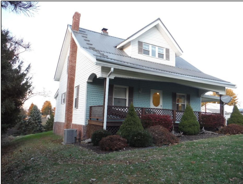
Photo 27 (9287), Haslam Farmstead (TT-004), Residence, 52017 Sykes Ridge Rd, Monroe County, Ohio, Northeast
