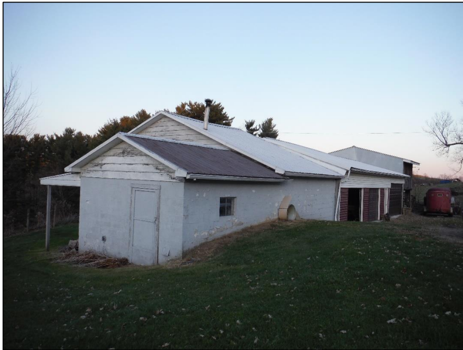
Photo 29 (9289), Haslam Farmstead (TT-004), Outbuildings, 52017 Sykes Ridge Rd, Monroe County, Ohio, East-Southeast
