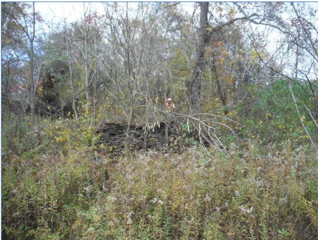
Photo 5.3-13 (Location 9009) Bank Barn Wall Outside Direct APE, Facing West.
