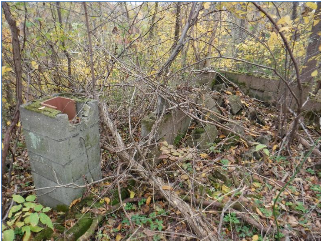
Photo 5.3-9 (Location 315) South Half of Foundation, Facing Southwest .
