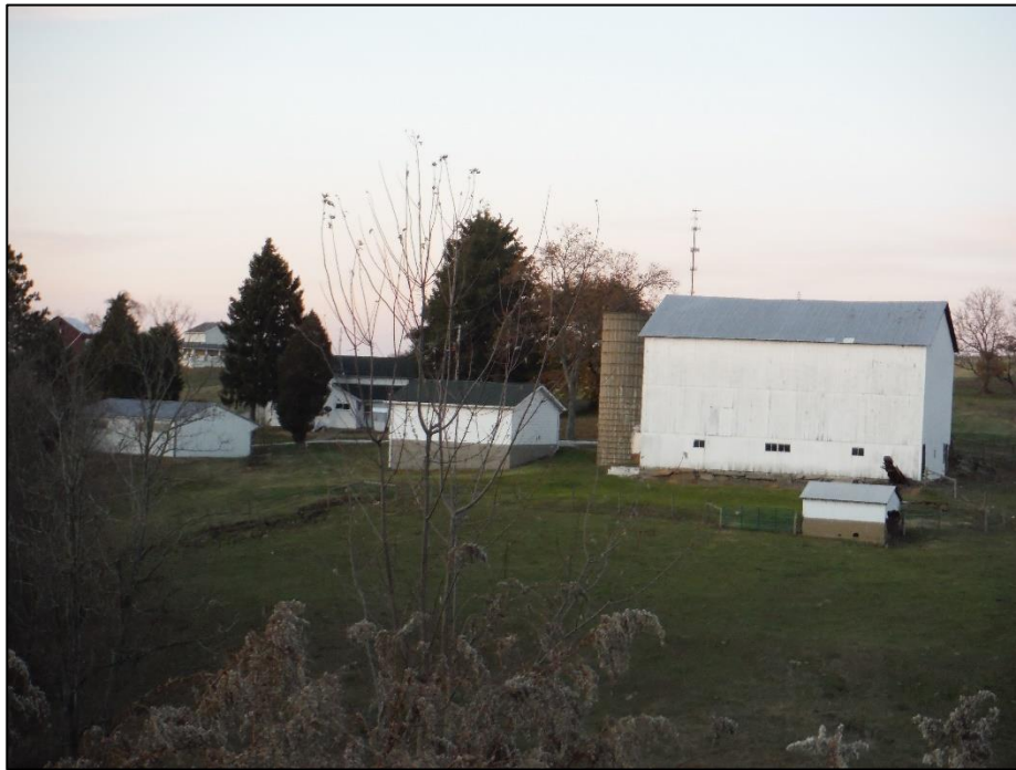
Photo 16 (9295), Rufener Farmstead (TT-003), Overview [(Left to Right) Modern Garage, Residence, Modern garage, Silo, Basement Barn, Pig Sty], 52067 Sykes Ridge Rd, Monroe County, Ohio, Northeast
