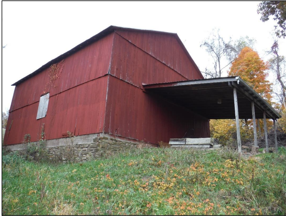
Photo 35 (8971), Blattler Residence and Barn (TT-005), Barn, 52246 Rouse Rd, Monroe County, Ohio, Southeast
