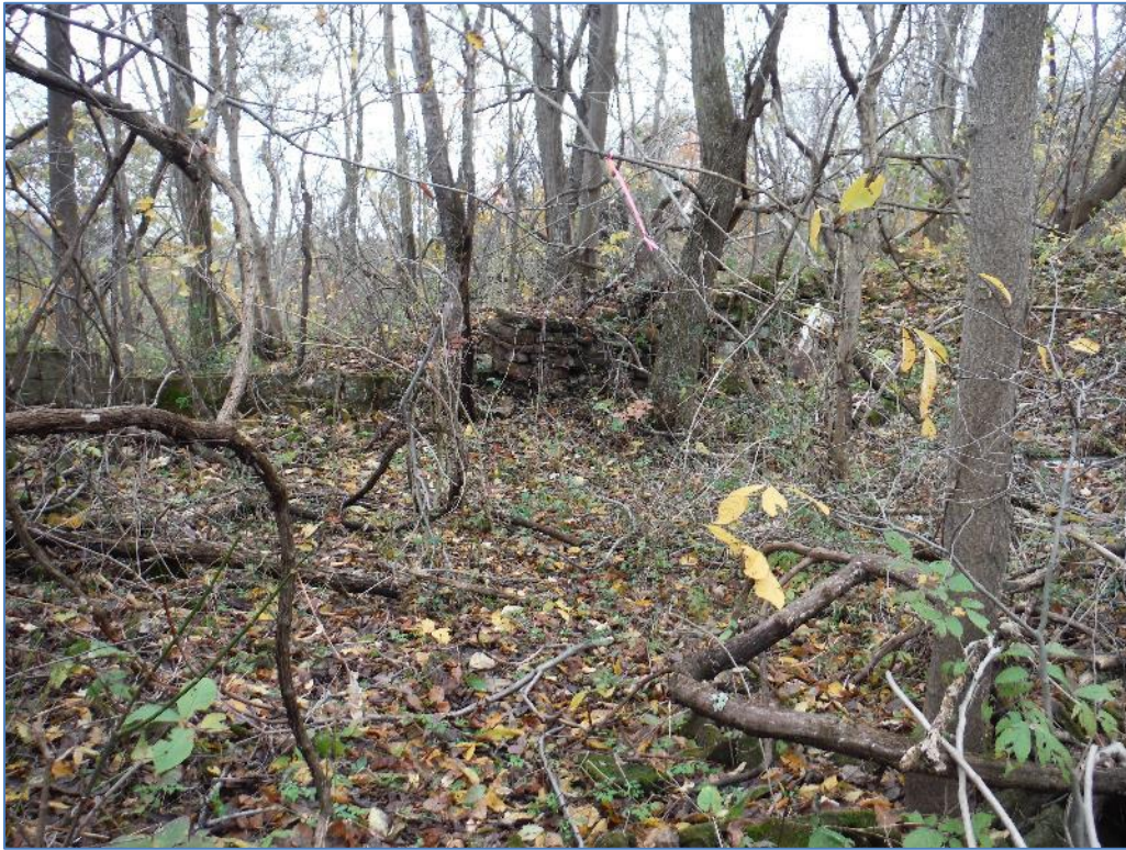
Photo 5.3-8 (Location 8991) North Half of Foundation, Facing West.
