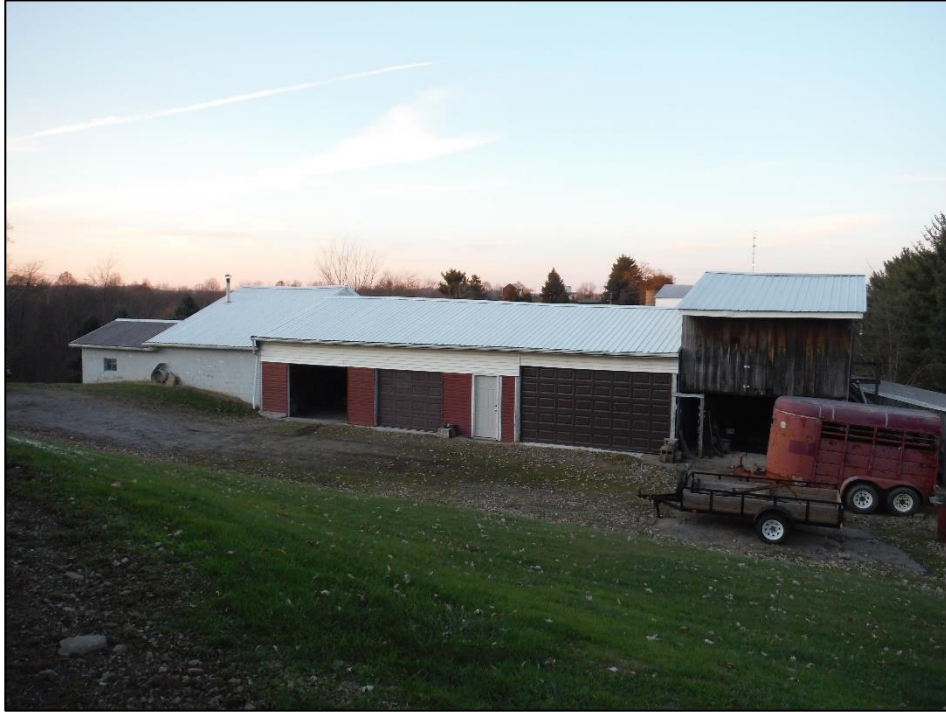
Photo 30 (9290), Haslam Farmstead (TT-004), Outbuildings, 52017 Sykes Ridge Rd, Monroe County, Ohio, Northeast
