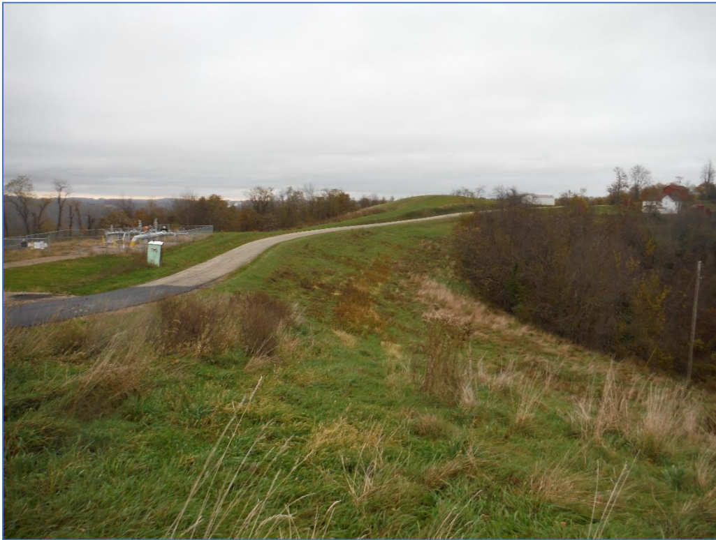
Photo 9185. Facing Northeast Showing Direct APE co-located with Existing Disturbance and Slope.
