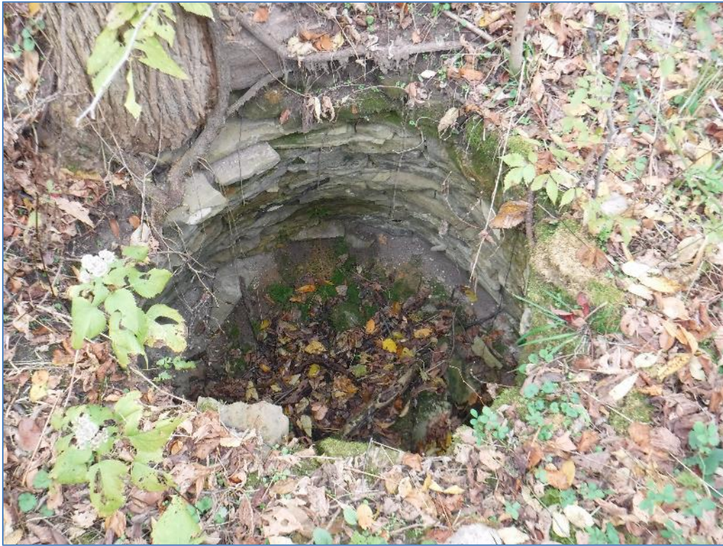
Photo 5.3-10 (Location 313) Well 1 West of House Foundation.
