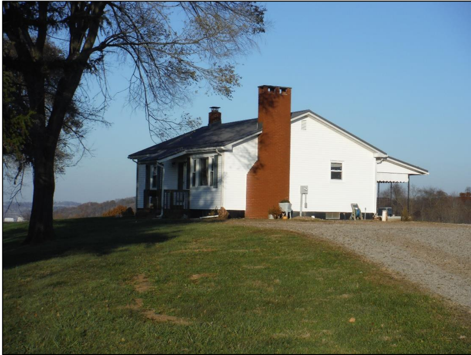
Photo 1 (9271), Lucas Farmstead (TT-001), Residence, 52189 Sykes Ridge Rd, Monroe County, Ohio, Northeast
