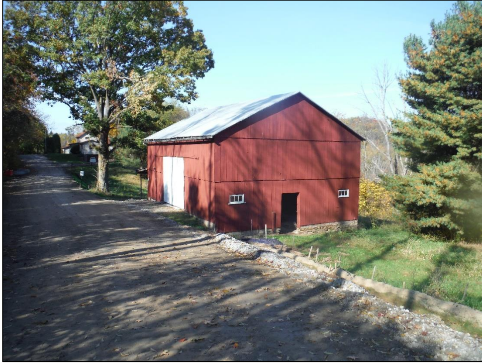
Photo 33 (8952), Blattler Residence and Barn (TT-005), Barn, 52246 Rouse Rd, Monroe County, Ohio, Northwest
