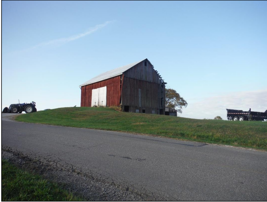
Photo 12 (8926), Deitrich Barn (TT-002), 52146 Sykes Ridge Rd, Monroe County, Ohio, West
