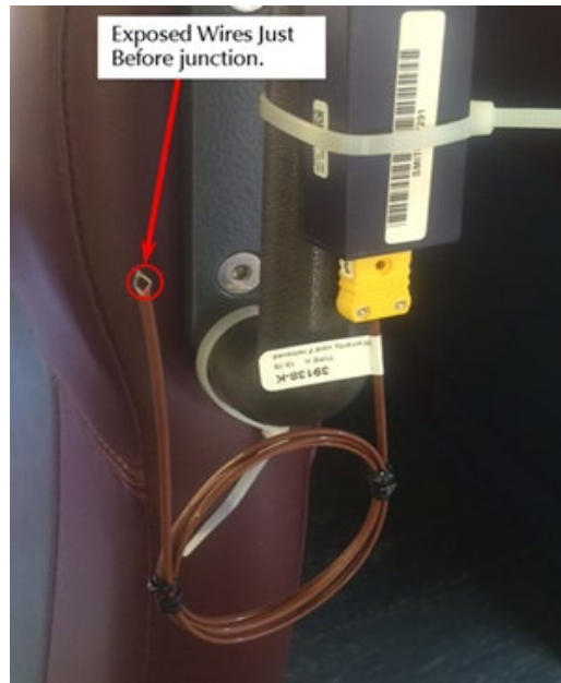
Figure 2-4. Thermocouple used for temperature measurement
