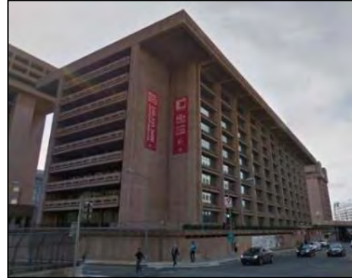
Figure 3-42 | Astral Building (Google Maps)
