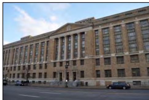
Figure 3-14 | USDA South Building
