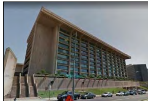
Figure 3-43 | Comsat Building (Google Maps)
