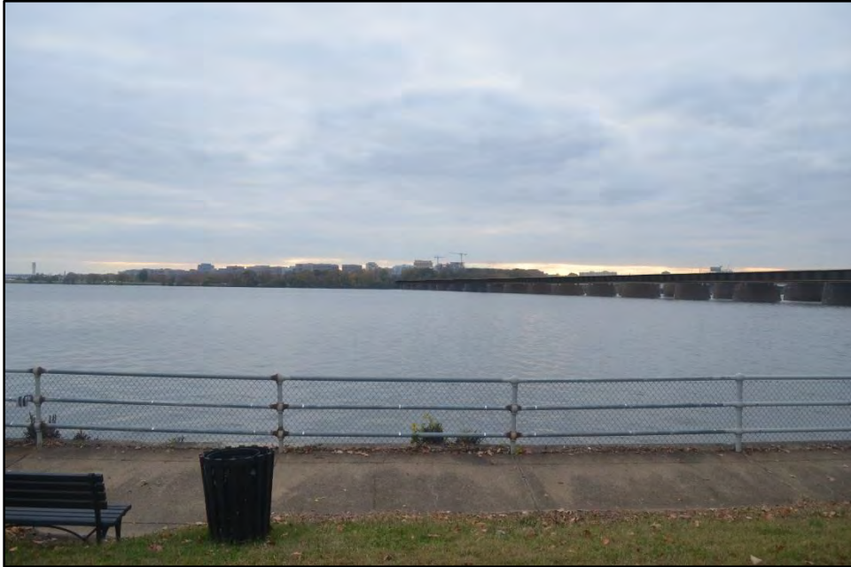
Action Alternative B: New railroad bridge visible.
