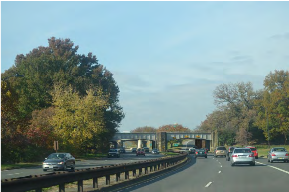
Action Alternative A: New railroad bridge abutment partially visible.
