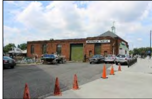
Figure 3-36 | Washington Marina Building
