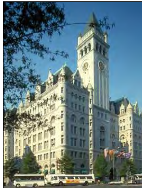
Figure 3-30 | The Old Post Office (National Park Service)
