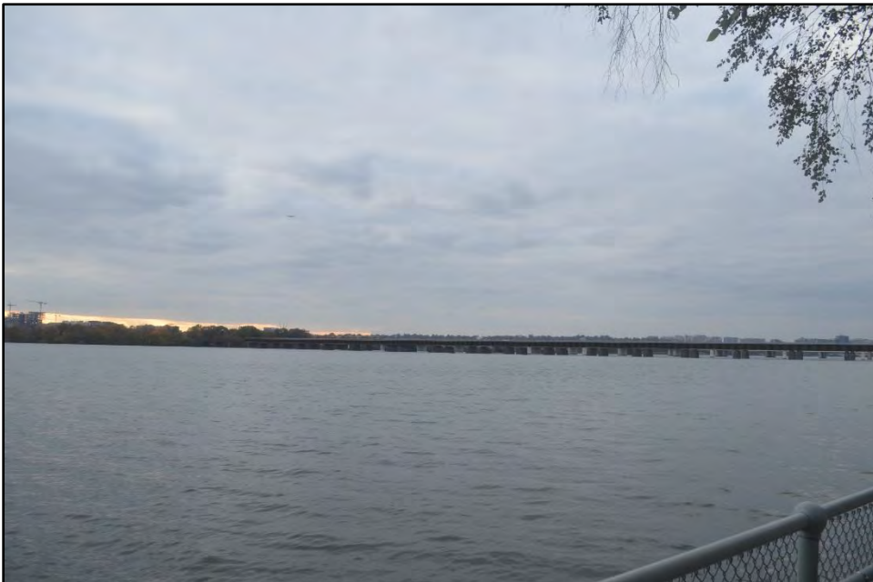
Action Alternative B: New railroad bridge visible.
