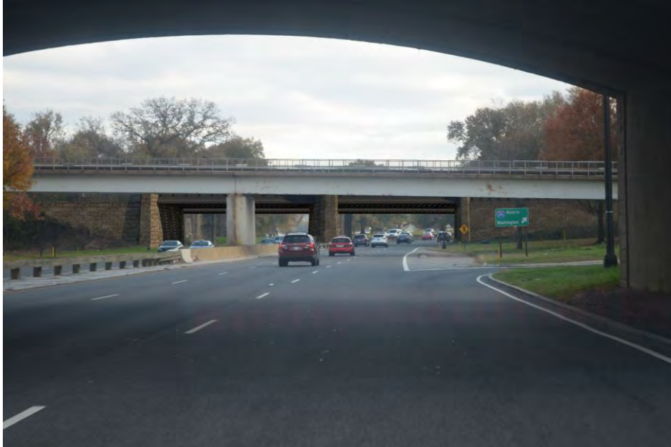
Action Alternative B: New railroad bridges visible behind Metrorail Bridge.
