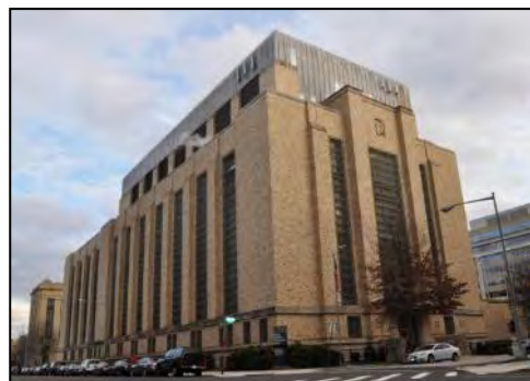
Figure 3-11 | Central Heating Plant
