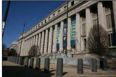
Figure 3-15 | BEP Main Building
