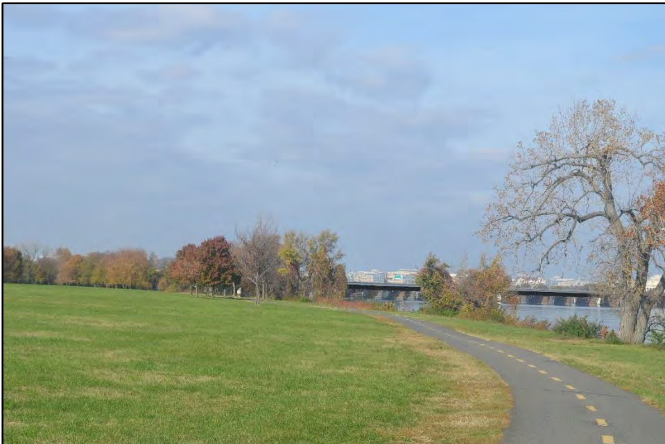
Action Alternative B: New railroad bridge visible.
