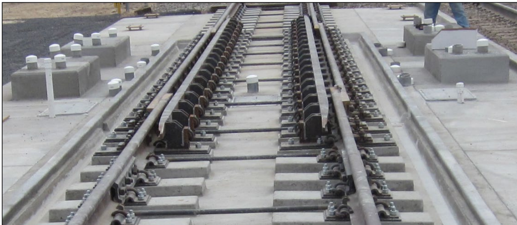
Figure 1. Gage Widened Section for Exposing the Wheel Tread for Ultrasonic Inspection
