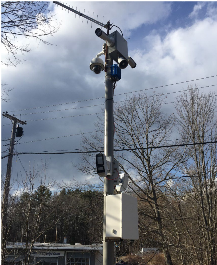
Figure 10 – Jordan Avenue Pole with Optex Sensors
