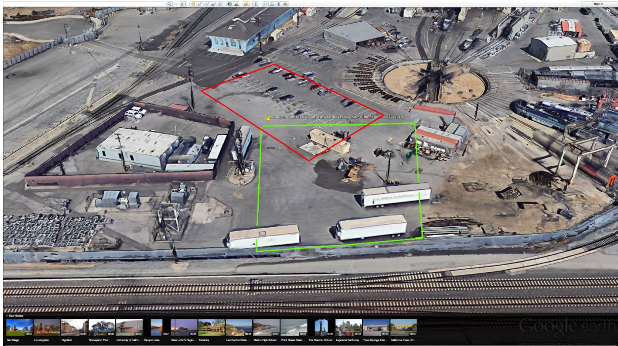
Figure 3. Amtrak’s Los Angeles Vehicle Maintenance Facility
