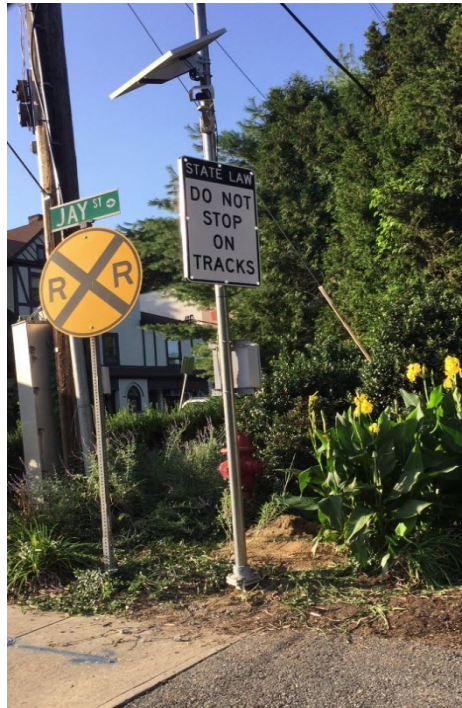
Figure 16. Laser-triggered, LED-enhanced, NYR9-5 sign
