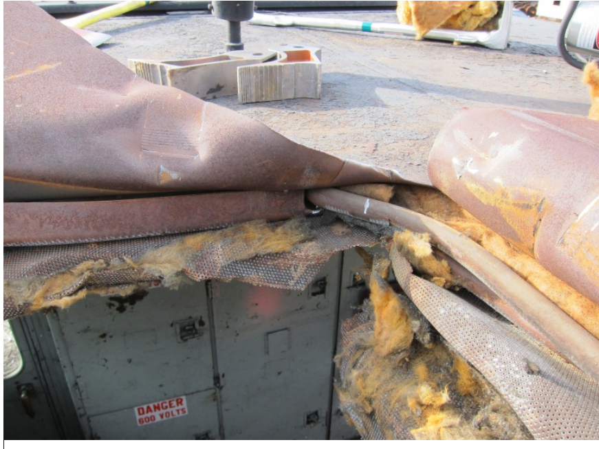
Figure 15: Roof Components, Including Insulation
