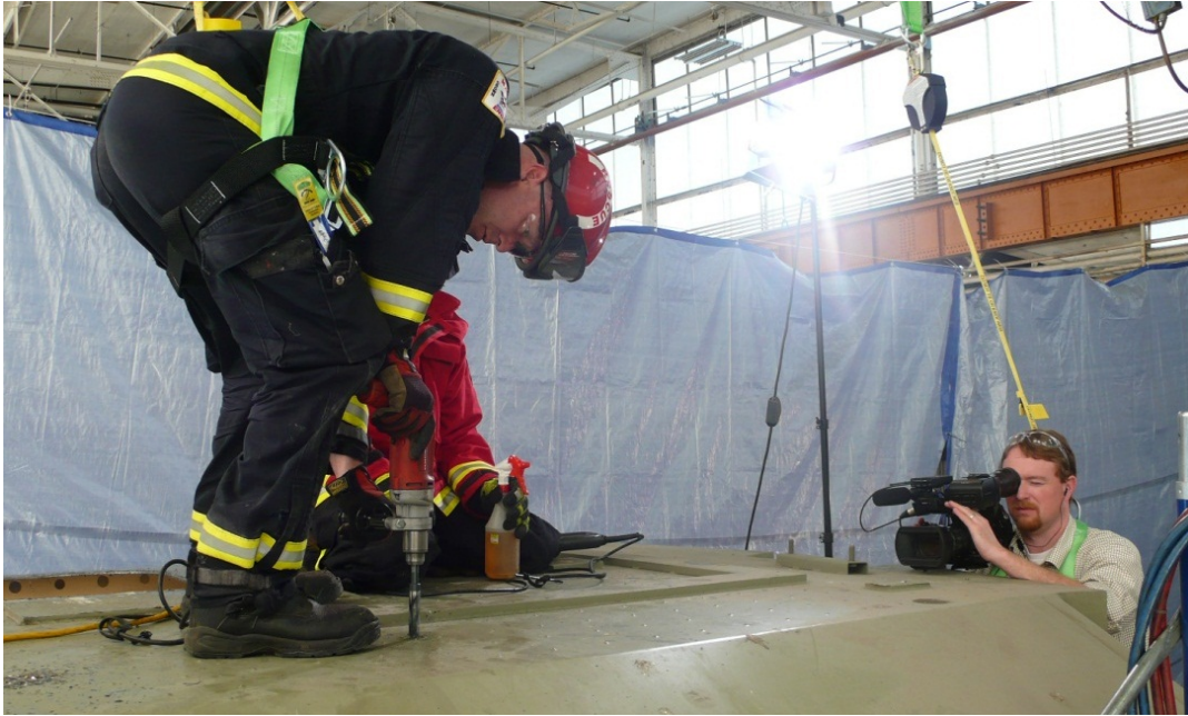
Figure 8: SD-70 Roof Access Demonstration
