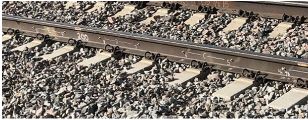
Figure 3. Friction welded studs attached to FAST track at TTC
