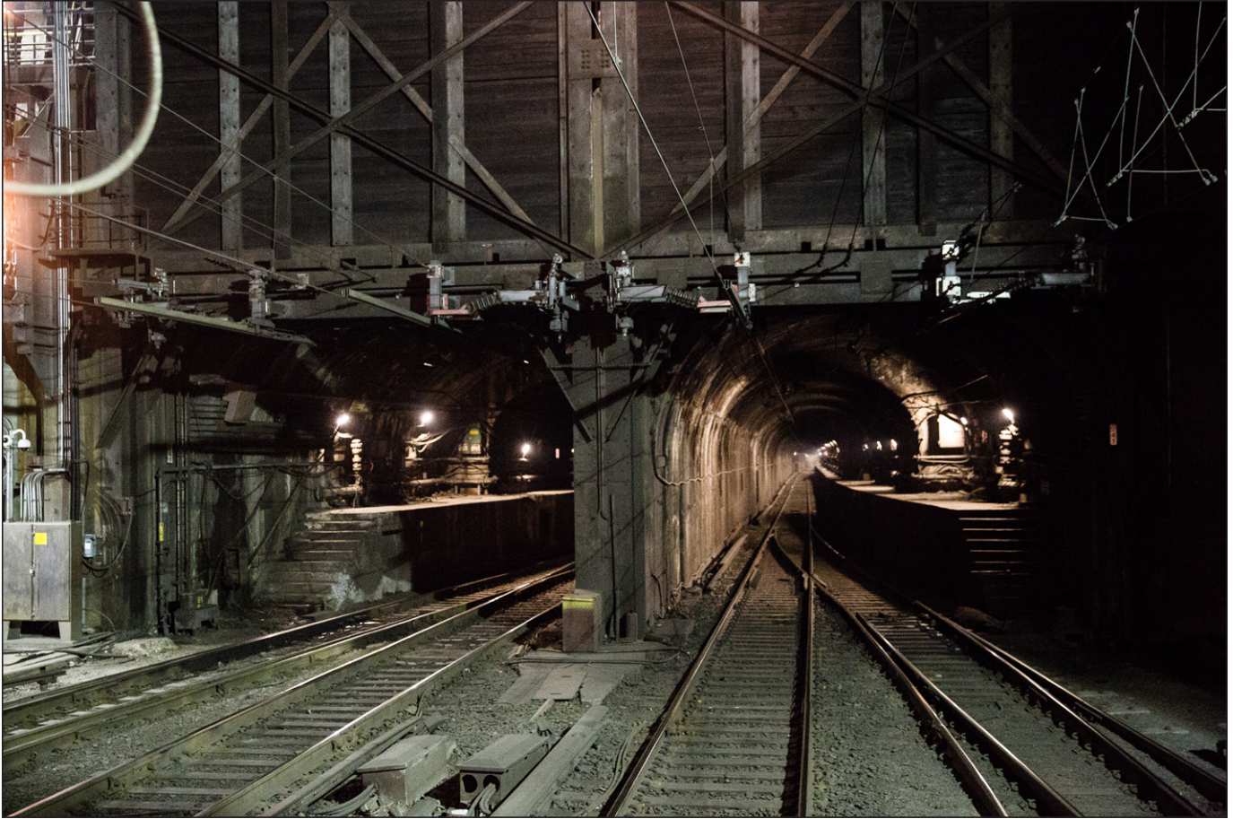
Entrance to the North River Tunnel in New York 1
