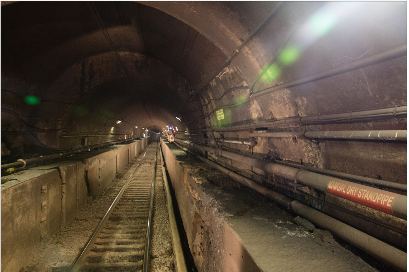
North River Tunnel showing damage including the bench walls and concrete lining
