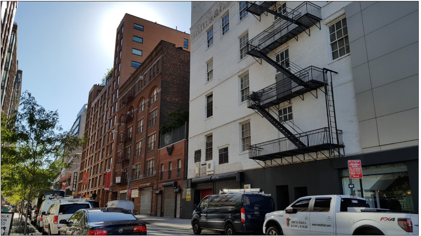
View of the south side of West 28th Street, east of Eleventh Avenue, 17 in the West Chelsea Historic District.
