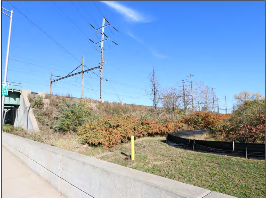
View northeast of the Northeast Corridor (NEC)/Pennsylvania Railroad (PRR) New York to Philadelphia Historic District at the southwest end of the APE in the Town of Secaucus.
