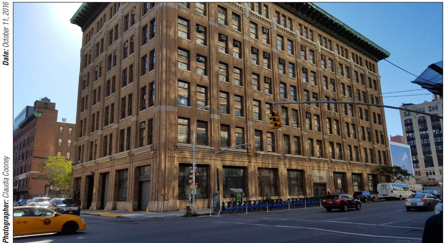
Otis Elevator Building in West Chelsea Historic District, 246-260 Eleventh Avenue. View southeast on Eleventh Avenue. 14
