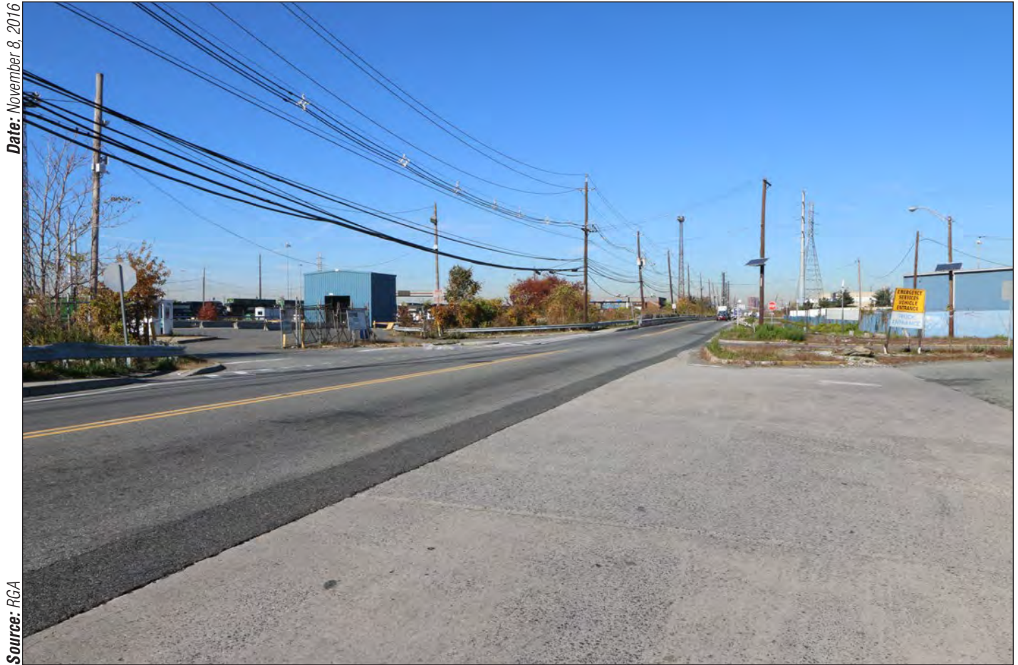
View northeast of County Road where it runs above the Jersey City Water Works Historic District in the Town of Secaucus, looking toward the NEC.
