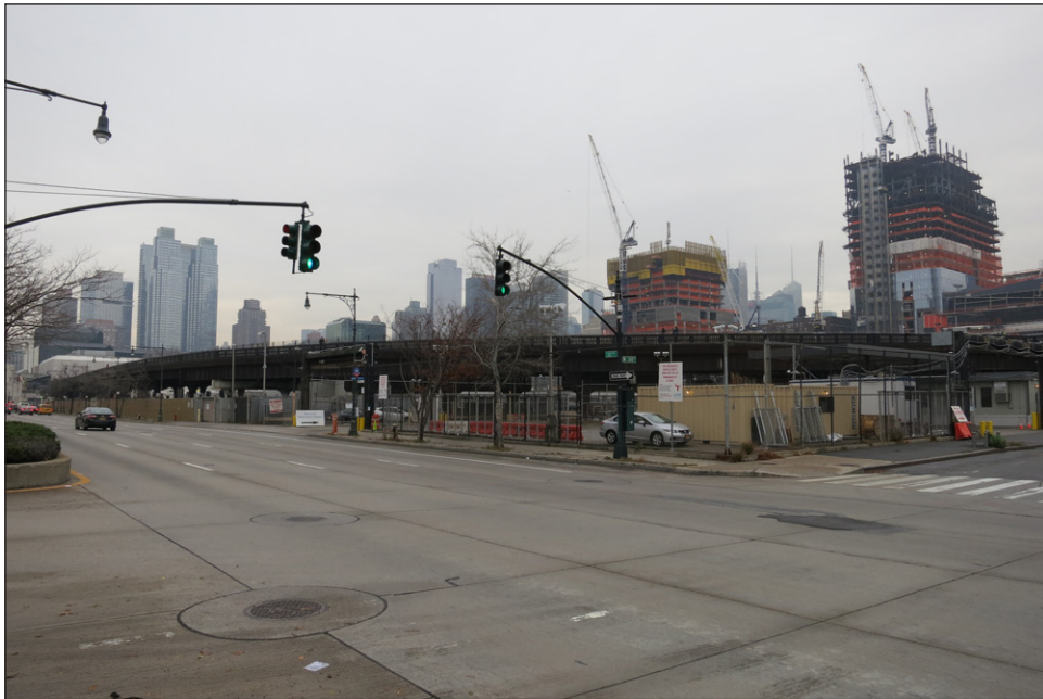
View northeast of the High Line at Twelfth Avenue and West 30th Street.
