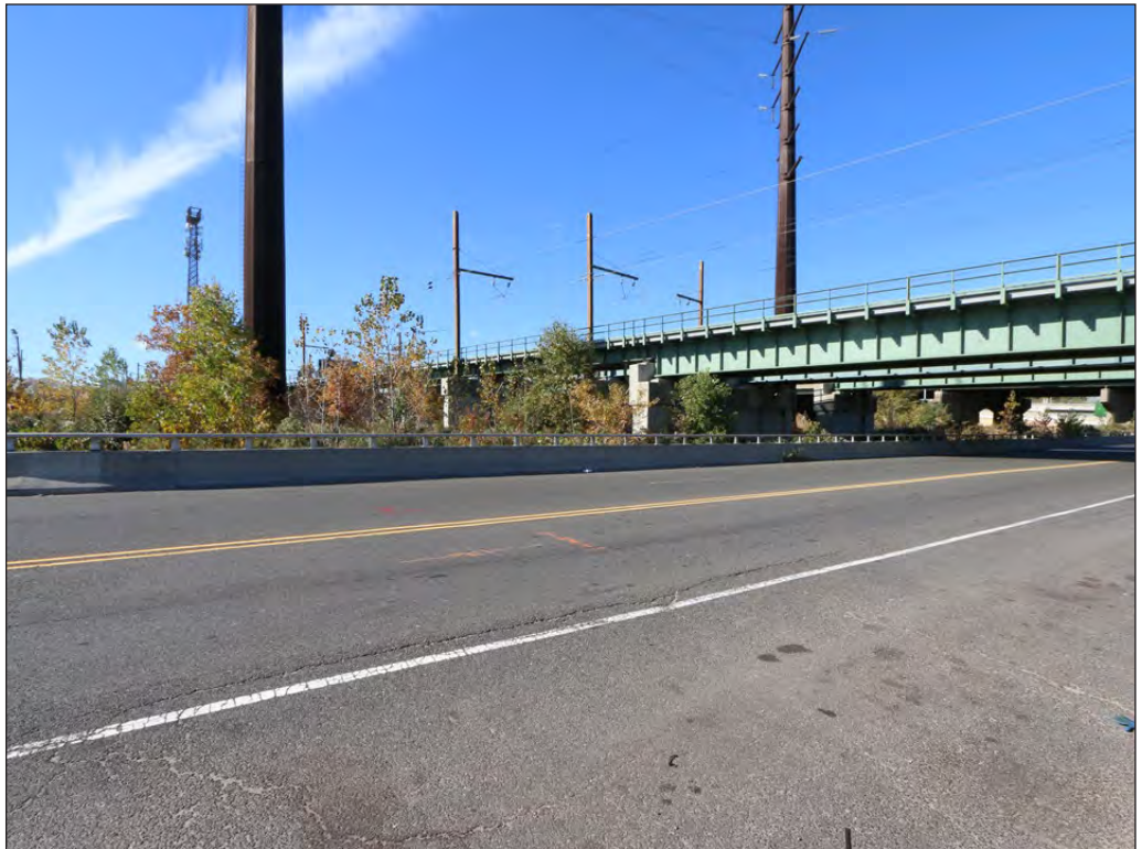
View west of the NEC/PRR Historic District at the southwest end of the APE, where it crosses over County Road and the Jersey City Water Works Historic District (below ground), in the Town of Secaucus.
