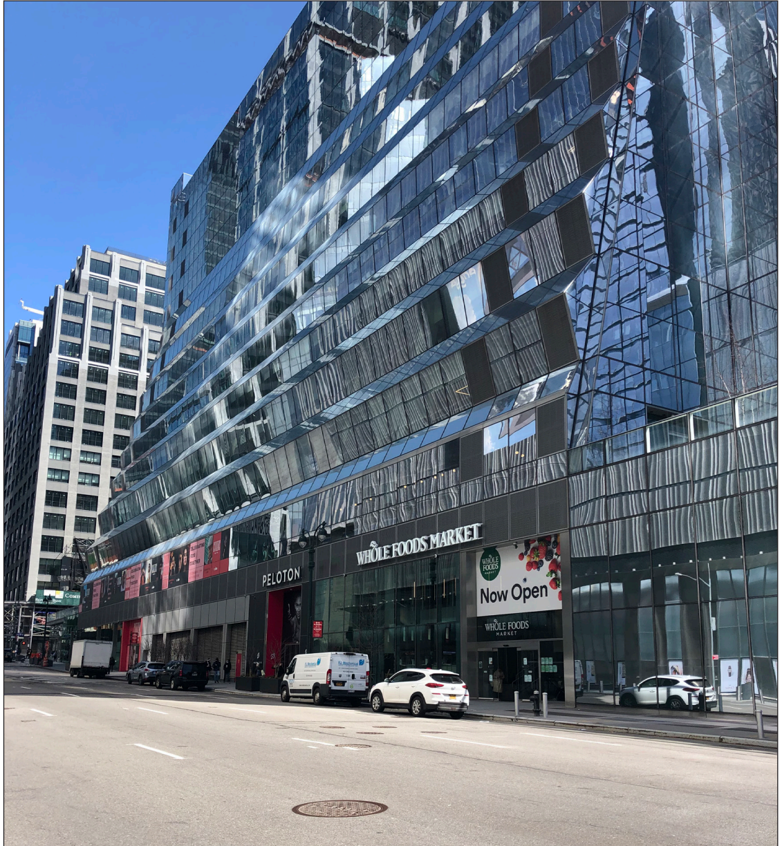
Building at 450 West 33rd Street 25
