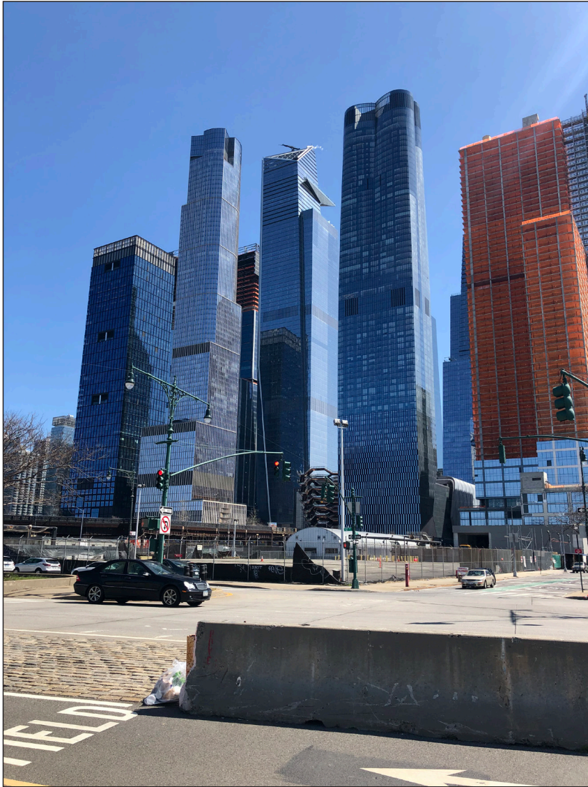
Corner of Twelfth Avenue and West 29th Street 16 from Hudson River Park, facing northeast
