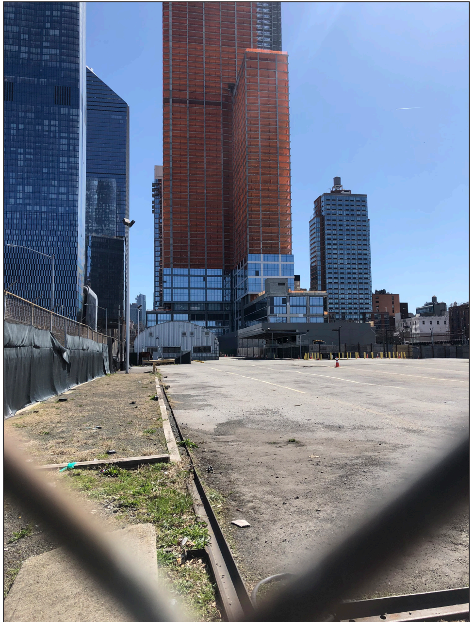
Twelfth Avenue Fan Plant site, facing east 18
