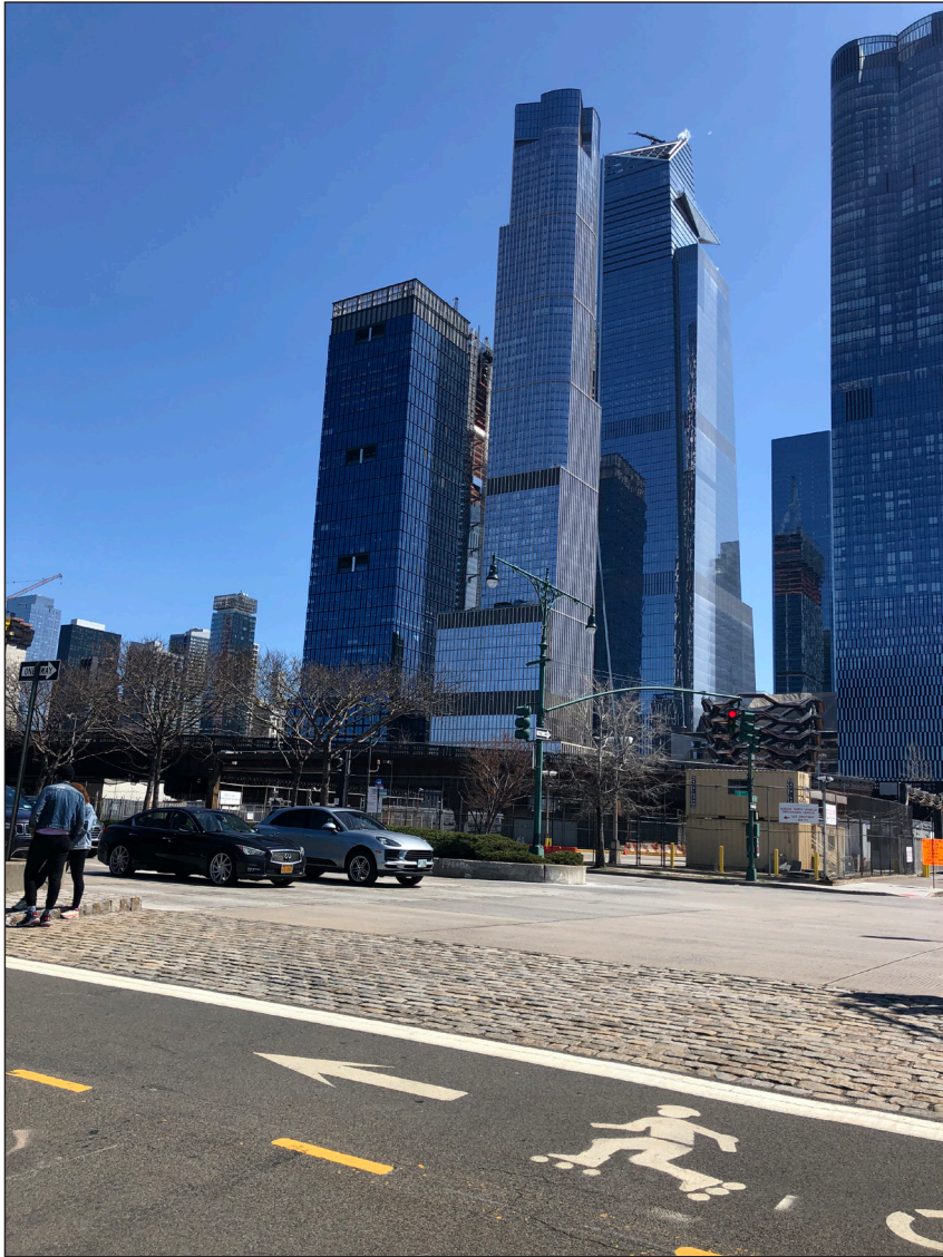
Hudson Yards Development with High Line in the foreground from Twelfth Avenue at West 30th Street, facing northeast 21
