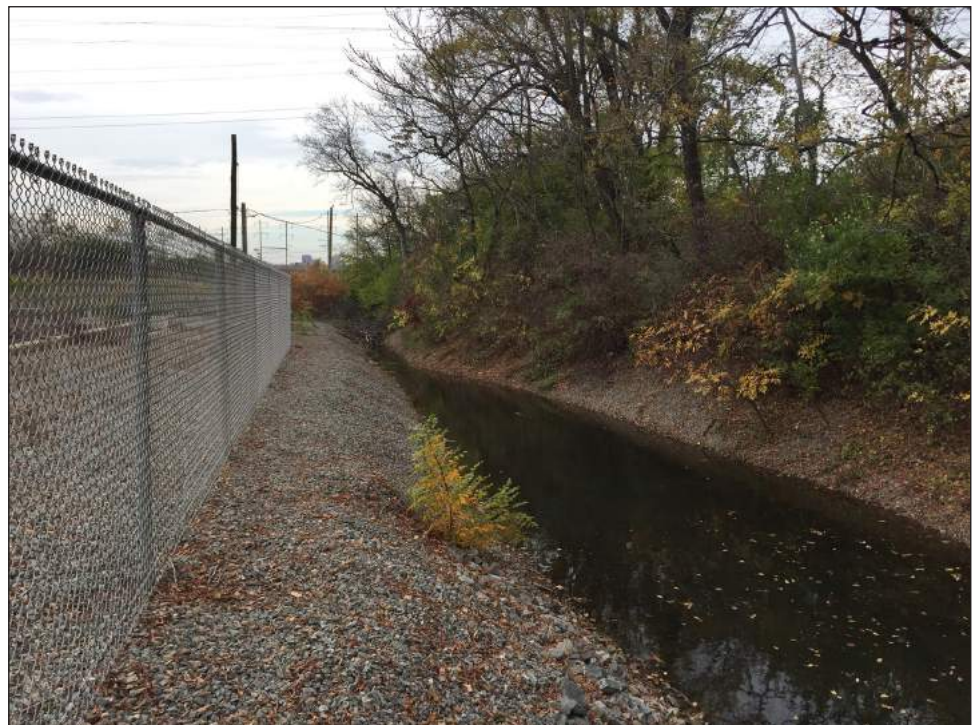
View of Detention Basin E, facing west. 4
