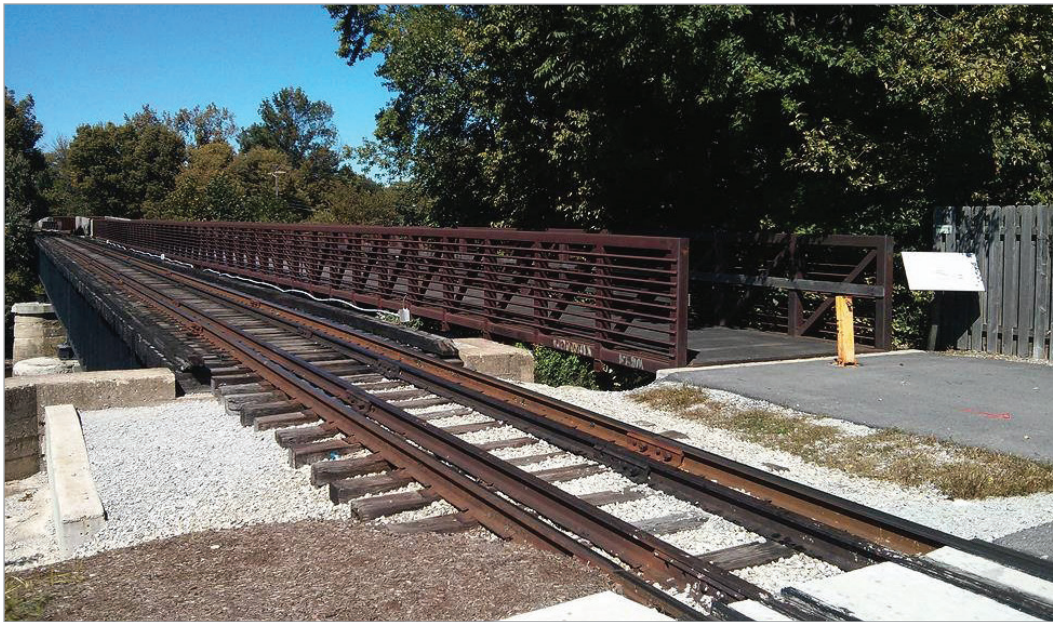
A trail bridge was built parallel to the rail bridge on the White River Greenway in Indiana. (Photo courtesy of the Rails-to-Trails Conservancy).
