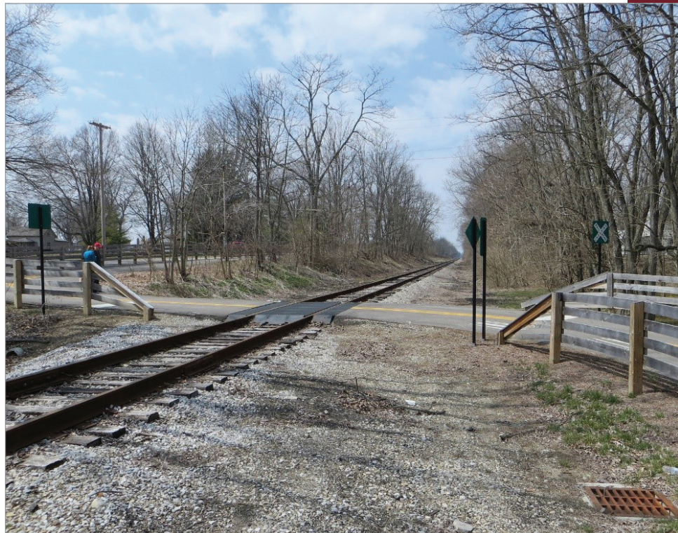
A trail/track crossing on the Camp Chase Trail in Ohio. The trail bends in order to cross the tracks at 90°. (Photo courtesy of the Rails-to-Trails Conservancy)
