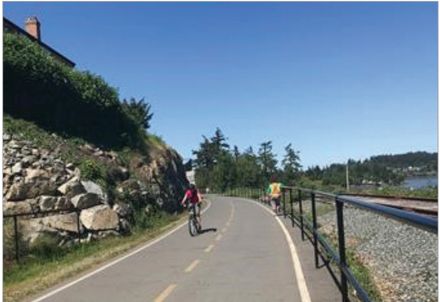
The E&N Rail Trail Humpback Connector on near Victoria, British Columbia. (Photo courtesy of Capital Regional District)
