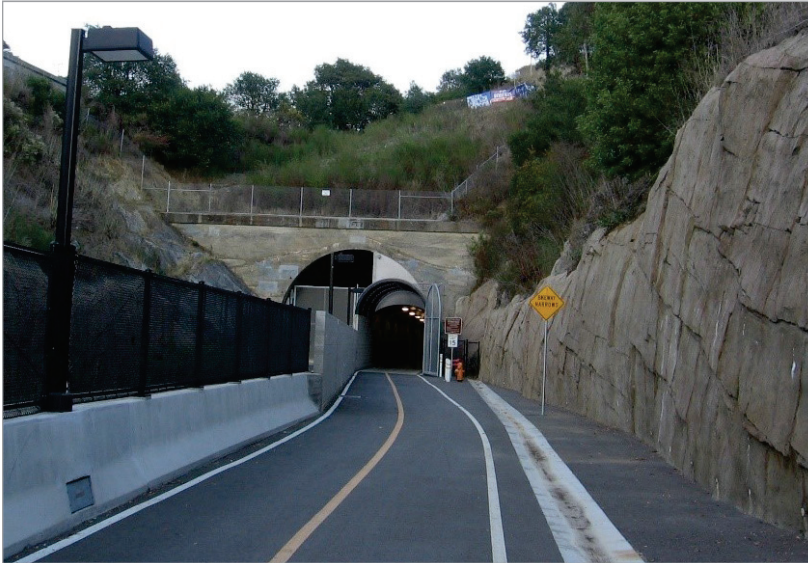
The shared-use Cal Park Hill Tunnel along the SMART commuter rail line in California (Photo courtesy of the Marin Independent Journal)
