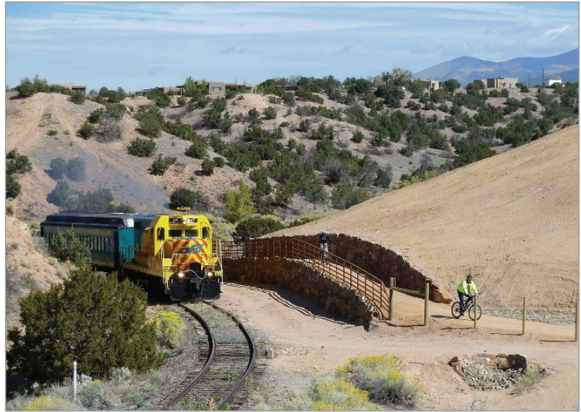
Vertical separation combined with a fence and retaining wall on the Santa Fe Trail in New Mexico. (Photo courtesy of Scott Belonger, P.E., Associate Principal for Loris and Associates)
