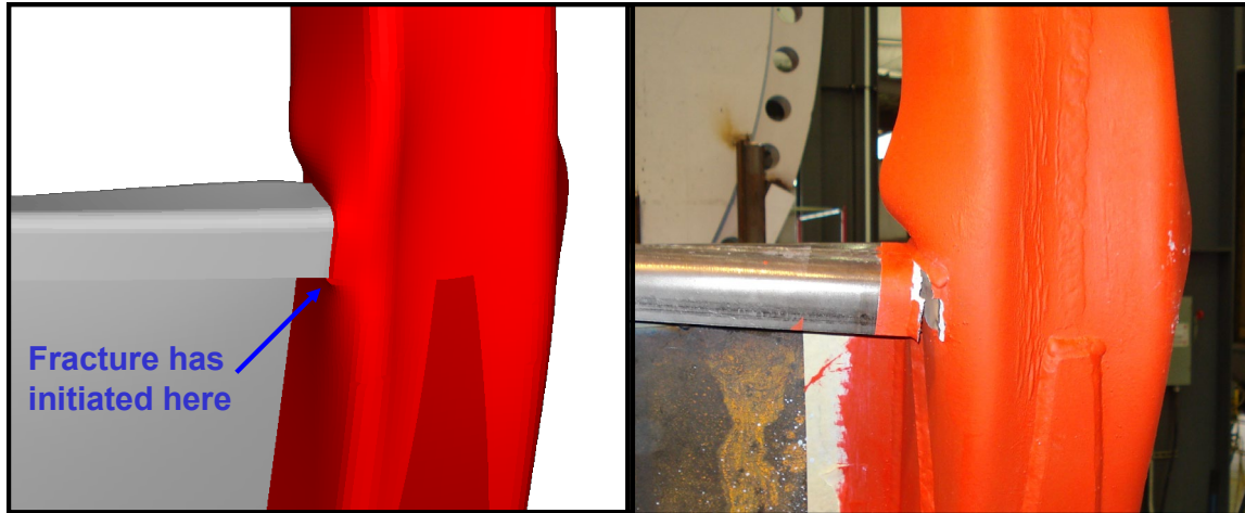
Figure 40. Comparison of predicted (left) and measured end frame deformation during corner post quasi-static crush test – detail showing back of corner post, opposite load application point
