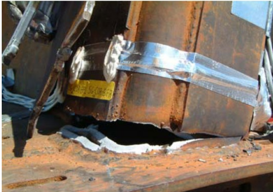
Figure D-10. Post-test photograph of base of corner post following coil impact
