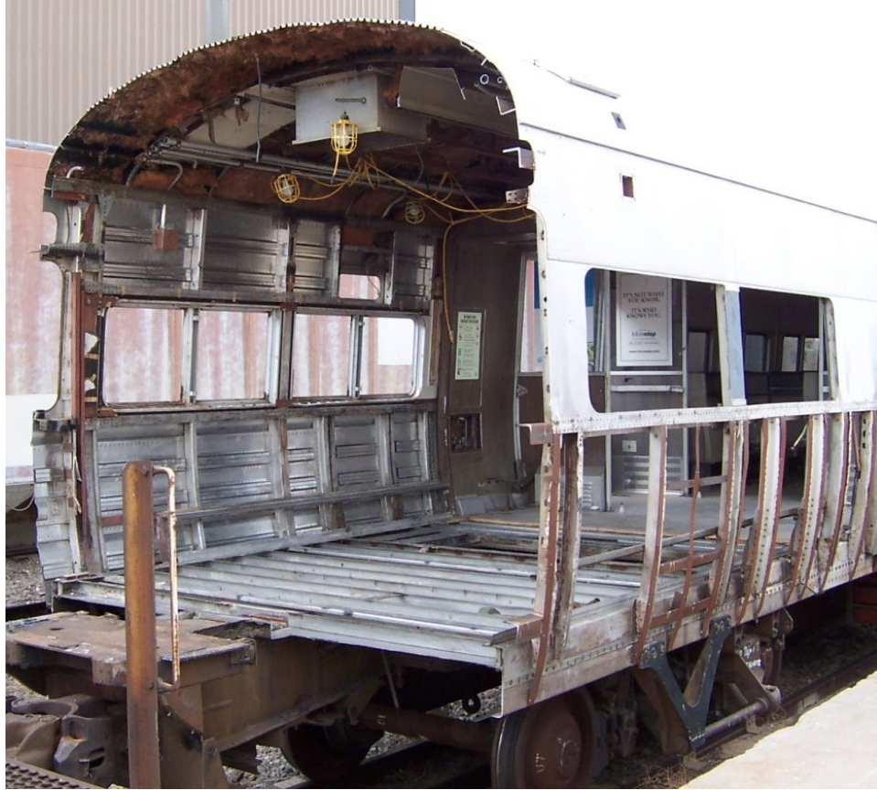
Figure 15. The cut M1 car ready for retrofit
