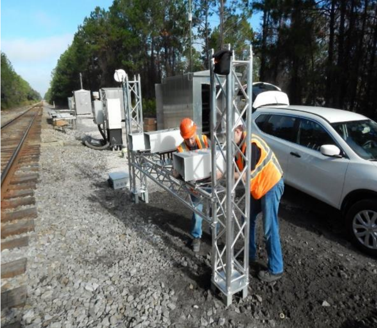
Figure 6. Installation of Axle-level Cameras at Hague Site
