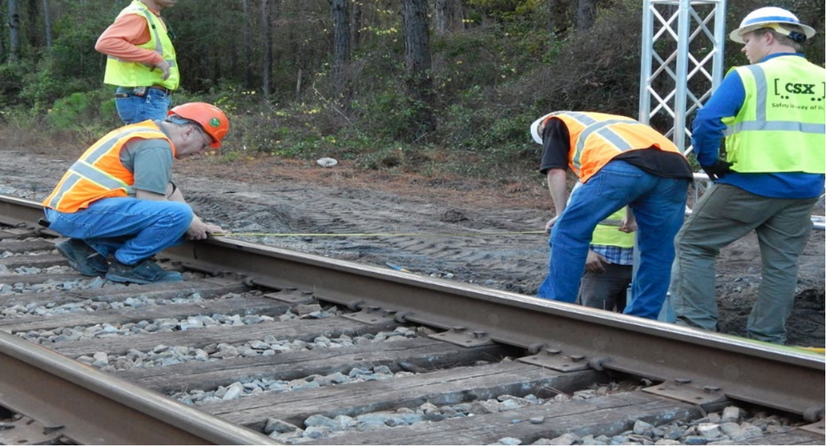
Figure 2. Installation Team Positioning Stanchions
