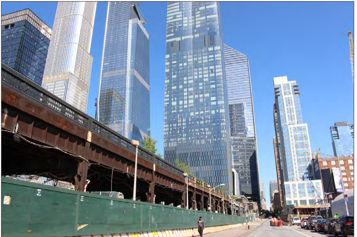
View to High Line, looking east on West 30th Street near Twelfth Avenue/Route 9A 2
