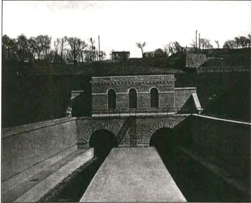
Figure 12a Hackensack Portals of Bergen Hill Tunnel (The New York Improvement and Tunnel Extension of the Pennsylvania Railroad p. 26.)
