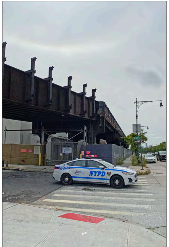
View south to High Line from Twelfth Avenue/Route 9A and West 33rd Street 4
