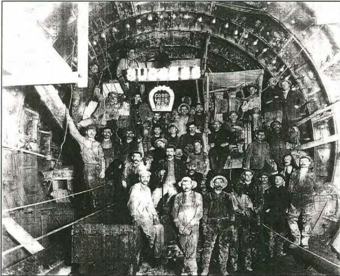
Figure 18 Front Street Long Island, "D" Line - Group of Workmen at Back of Trailing Platform Where Tunnels Meet, February 21 th 1908 (The Smithsonian Institution, National Museum of American History, Archives Center - Catalog # 80.0032.0000 - Photo 2077.)
