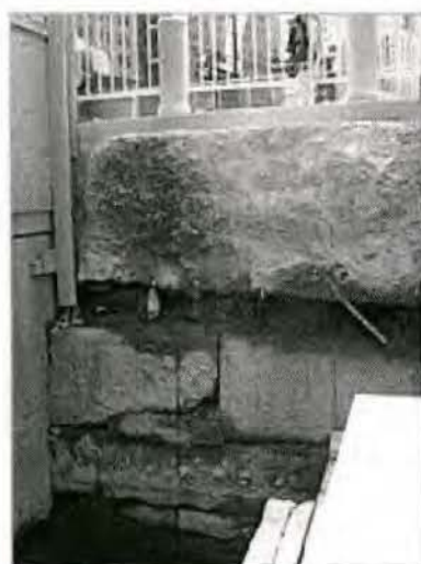
Port Authority of New York and New Jersey Newly exposed granite blocks from the historic river wall that lies just west of the World Trade Center site.
