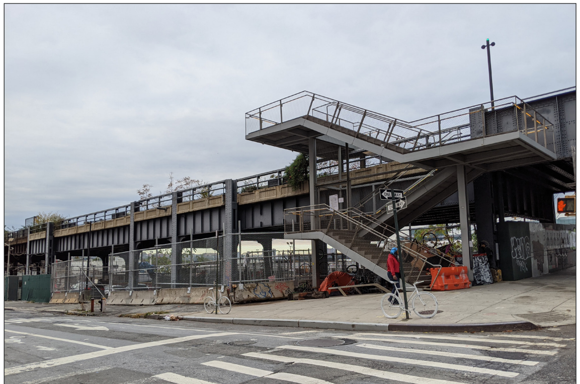
Project Site, view northwest at Eleventh Avenue and West 30th Street 6
