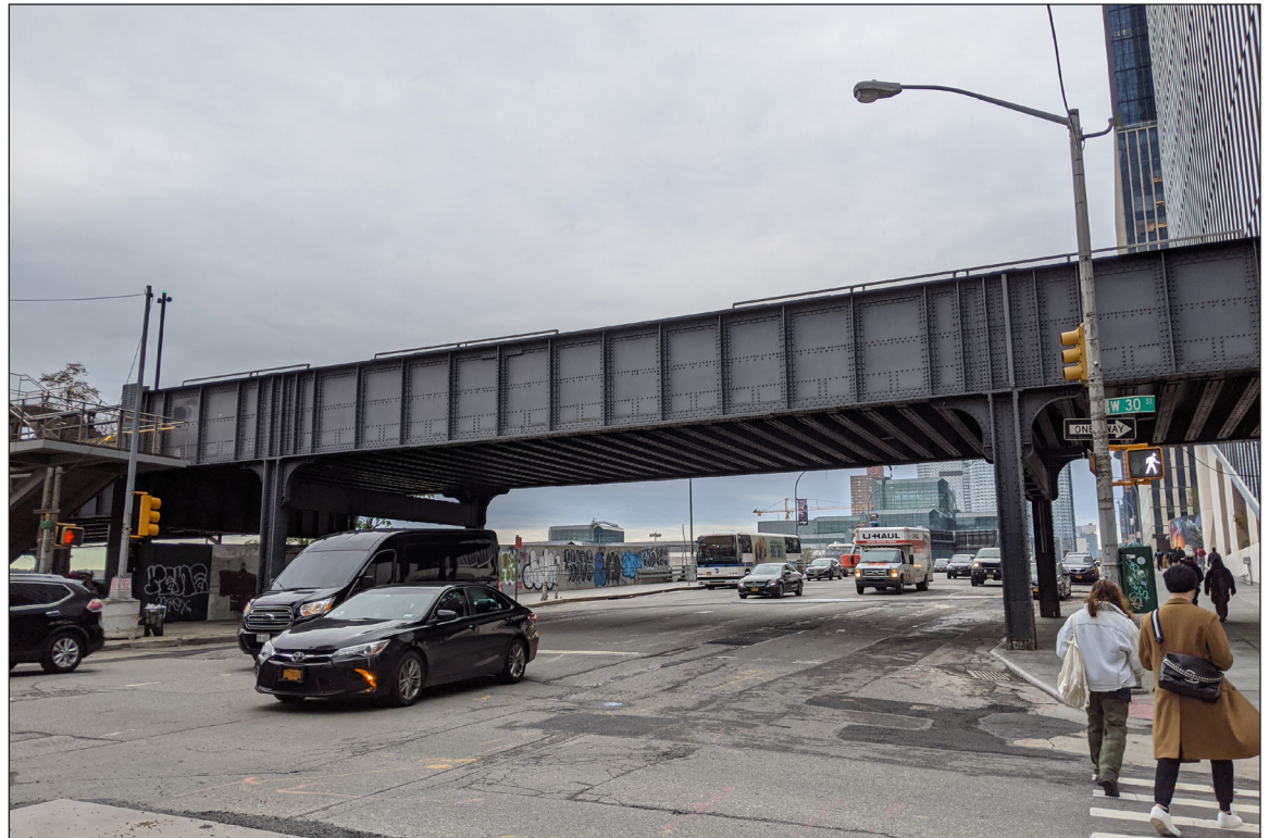
Project Site, view north on Eleventh Avenue from West 30th Street 7
