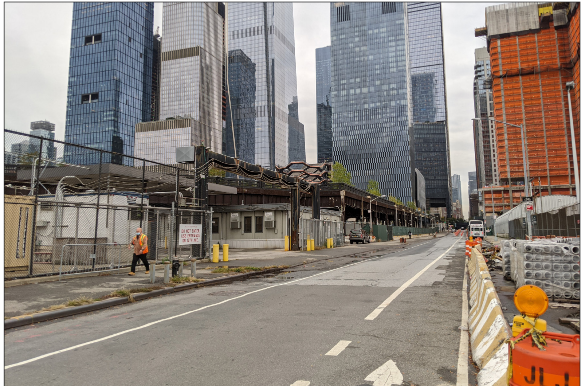
Project Site, view east on West 30th Street 5
