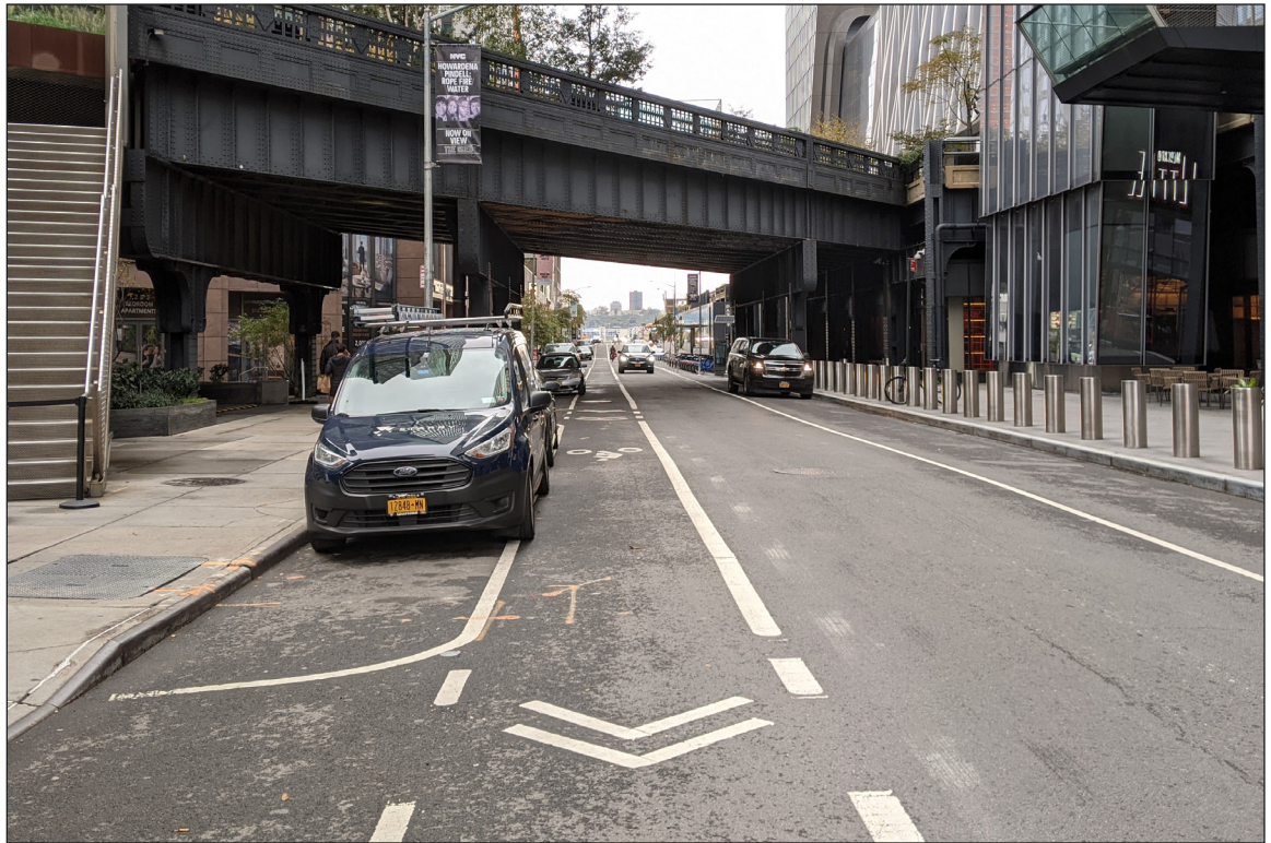
View west on West 30th Street adjacent to Hudson Yards 18
