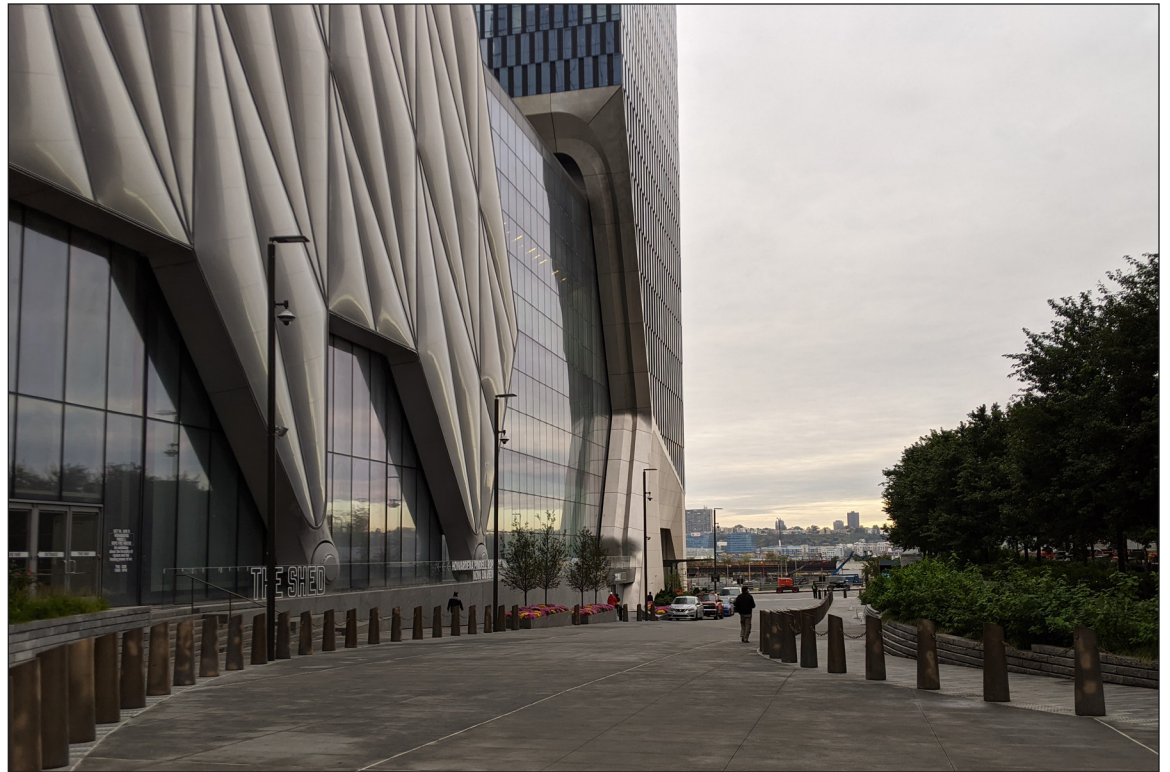
Hudson Yards, view west along service drive adjacent to the Shed 22
