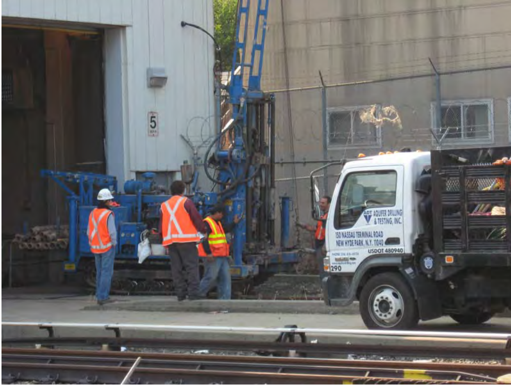
Picture 5 – (09/22/08) – Active test borings being conducted east of the Site during the Site-walk.
