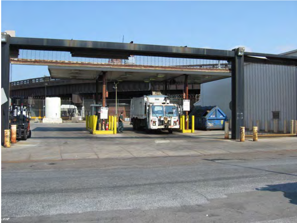
Picture 15 – (09/22/08) – Garbage truck filling station on southwestern corner of Site.
