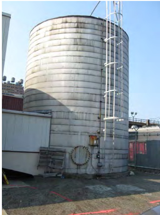
Picture 4 – (09/22/08) – Large AST holding water near the fire pump house on the southern portion of the Site.
