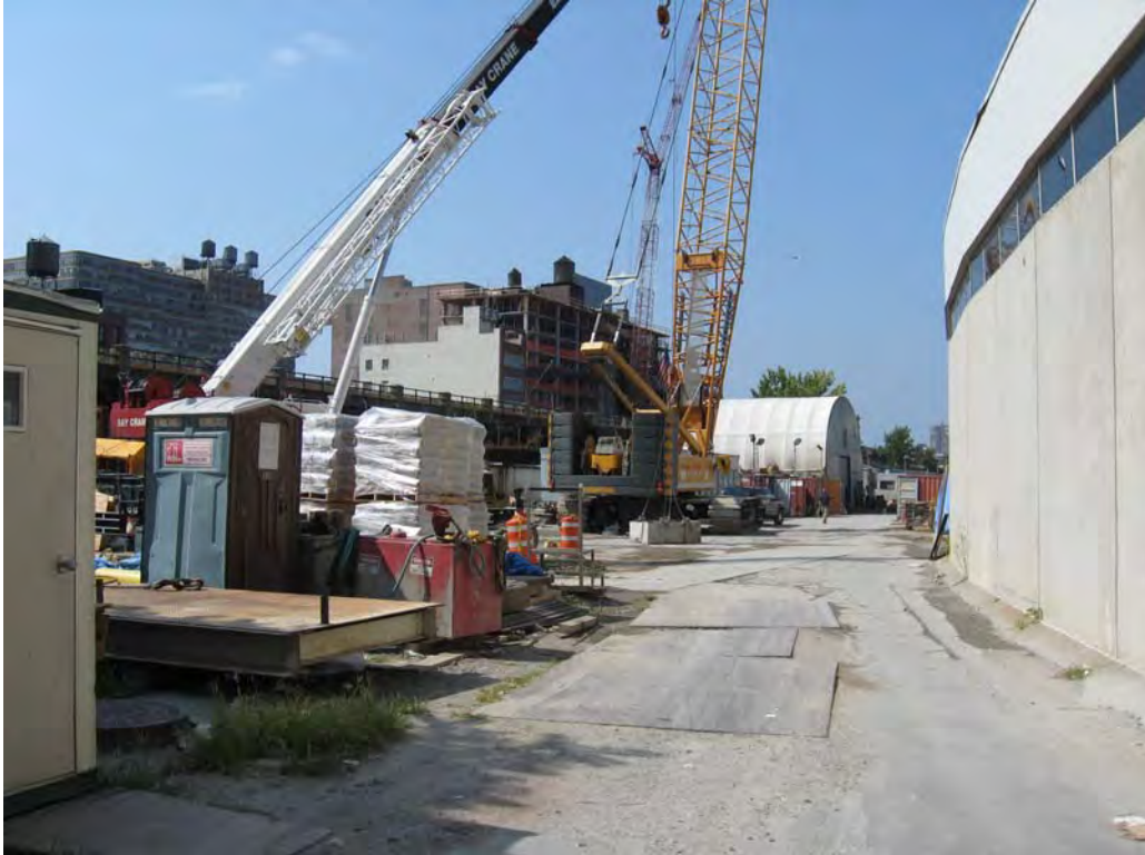
Picture 9 – (09/22/08) – Active construction site directly east of Site, facing west.
