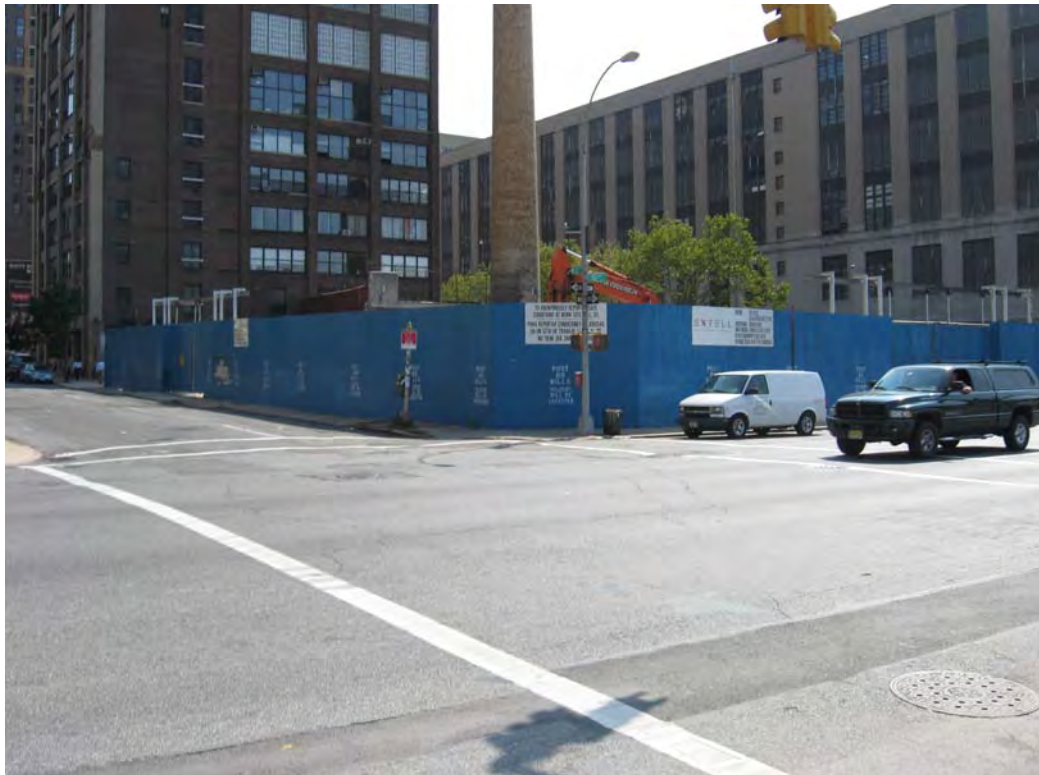
Picture 12 – (09/22/08) – Active construction site east of Site, east of 10 th Avenue.
