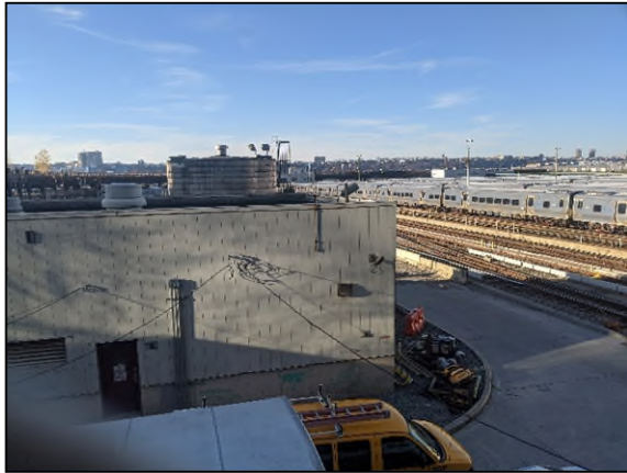
Photograph 1. View of southeastern portion of the Property on Lot 1, facing northwest.
