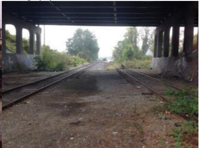
Railroad right-of-way under I-393 overpass
