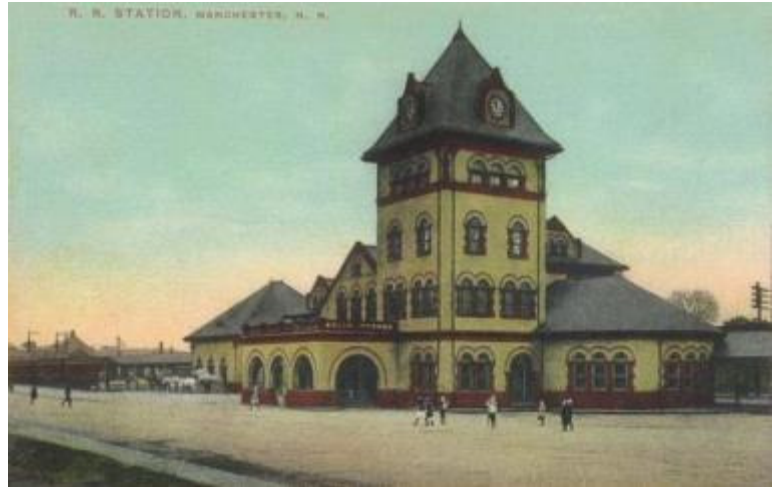
Figure 6-14: Historic Manchester Rail Station
