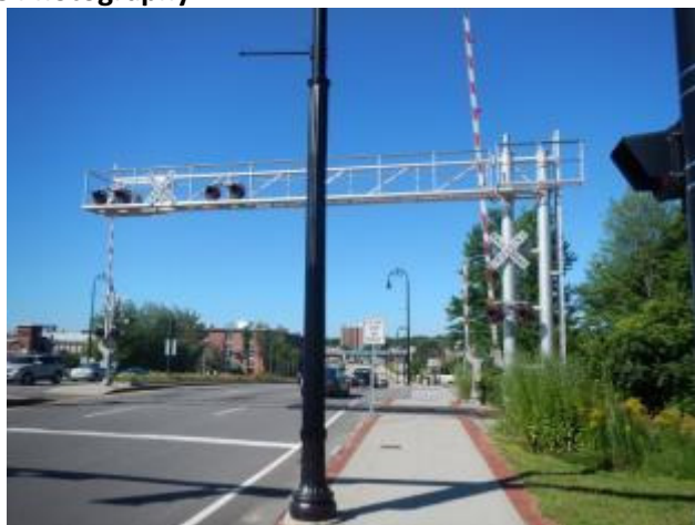
Facing west towards I-293
