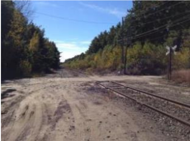
Hills Ferry Road at-grade crossing
