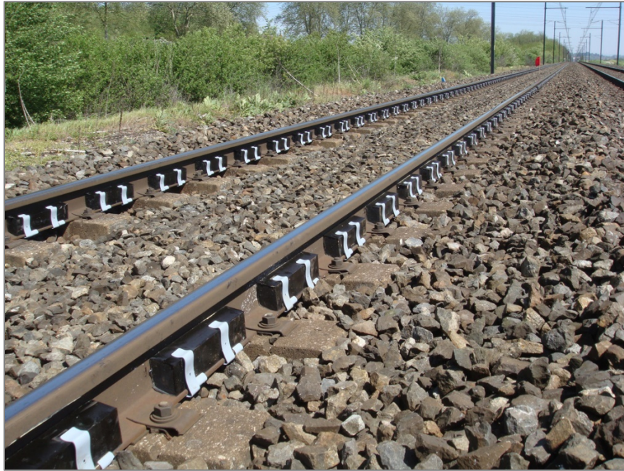
Figure 48: Tuned Rail Dampers
