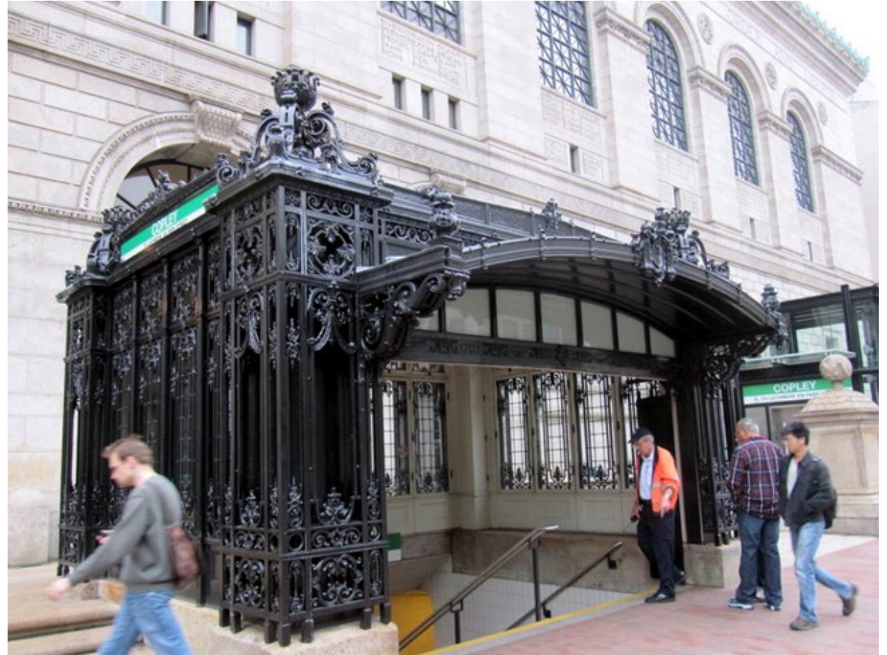
Photo Credit: APTA Committee, John Smatlak
