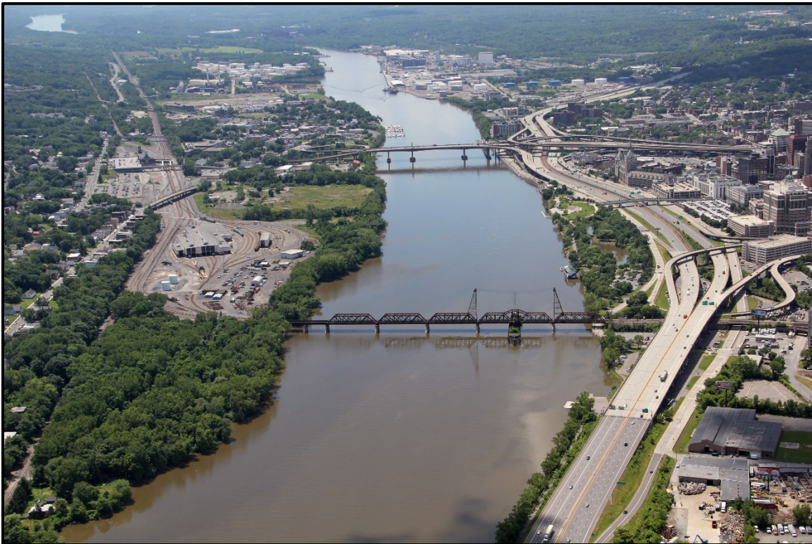
Photo C.2: LAB Elevation, Looking South (Dunn Memorial Bridge in Background)
