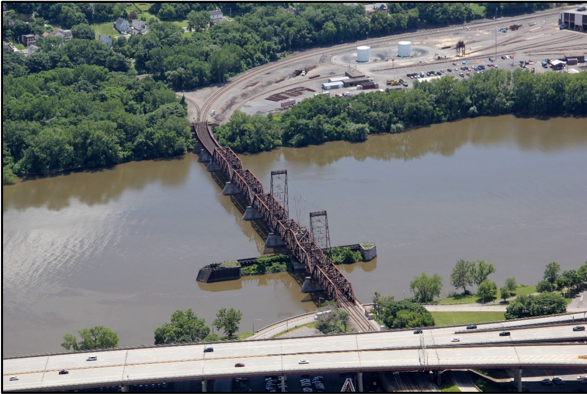
Photo C.3: LAB Looking East (Amtrak Maintenance Yard in Background)
