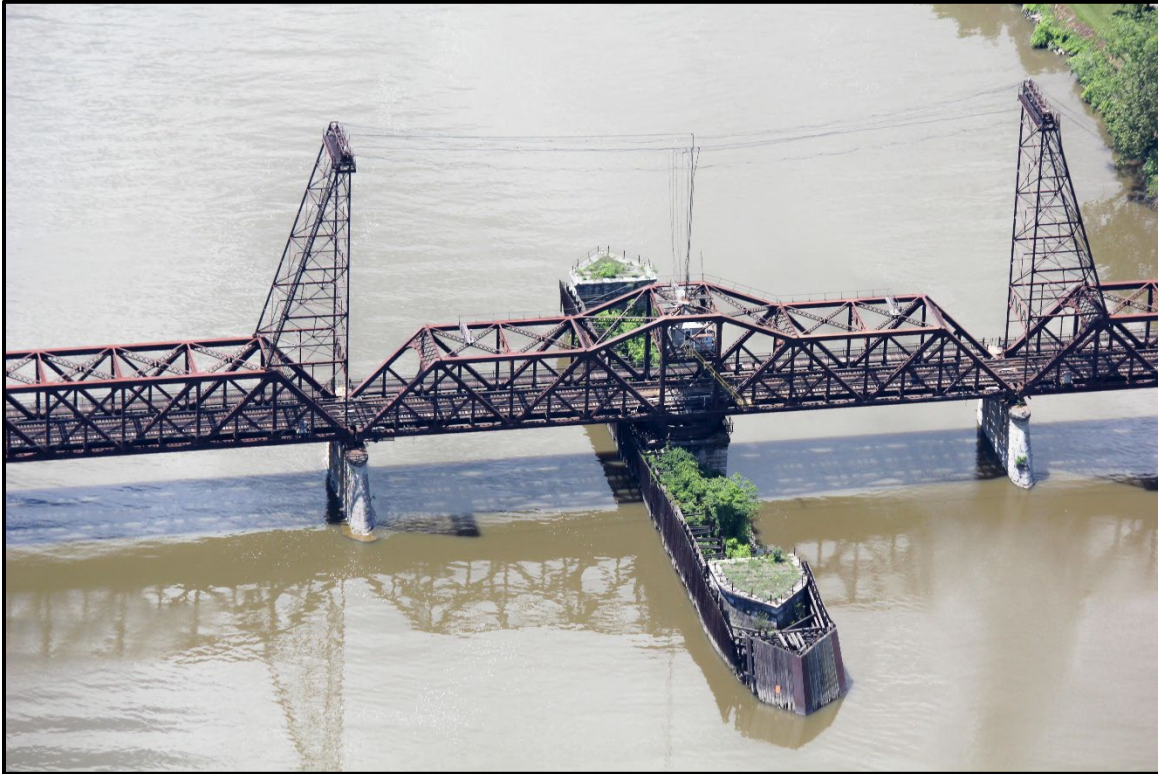
Photo C.1: LAB Swing Span Elevation, Looking South
