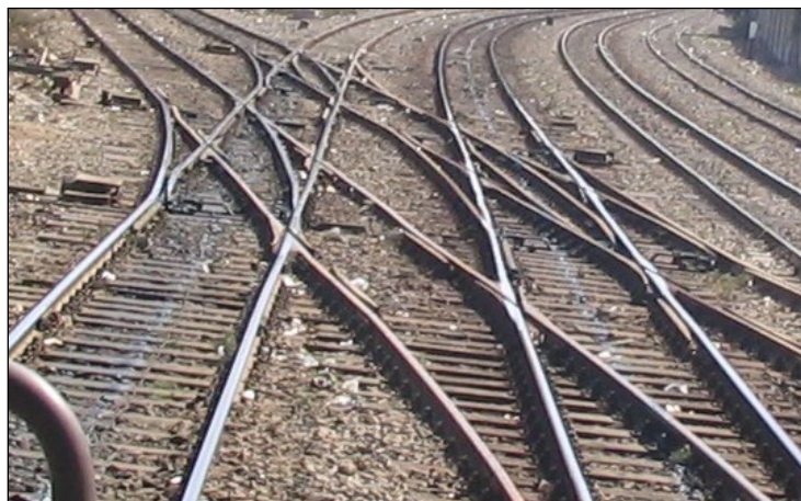
Figure A-2.14. Illustration of Slip Switches
