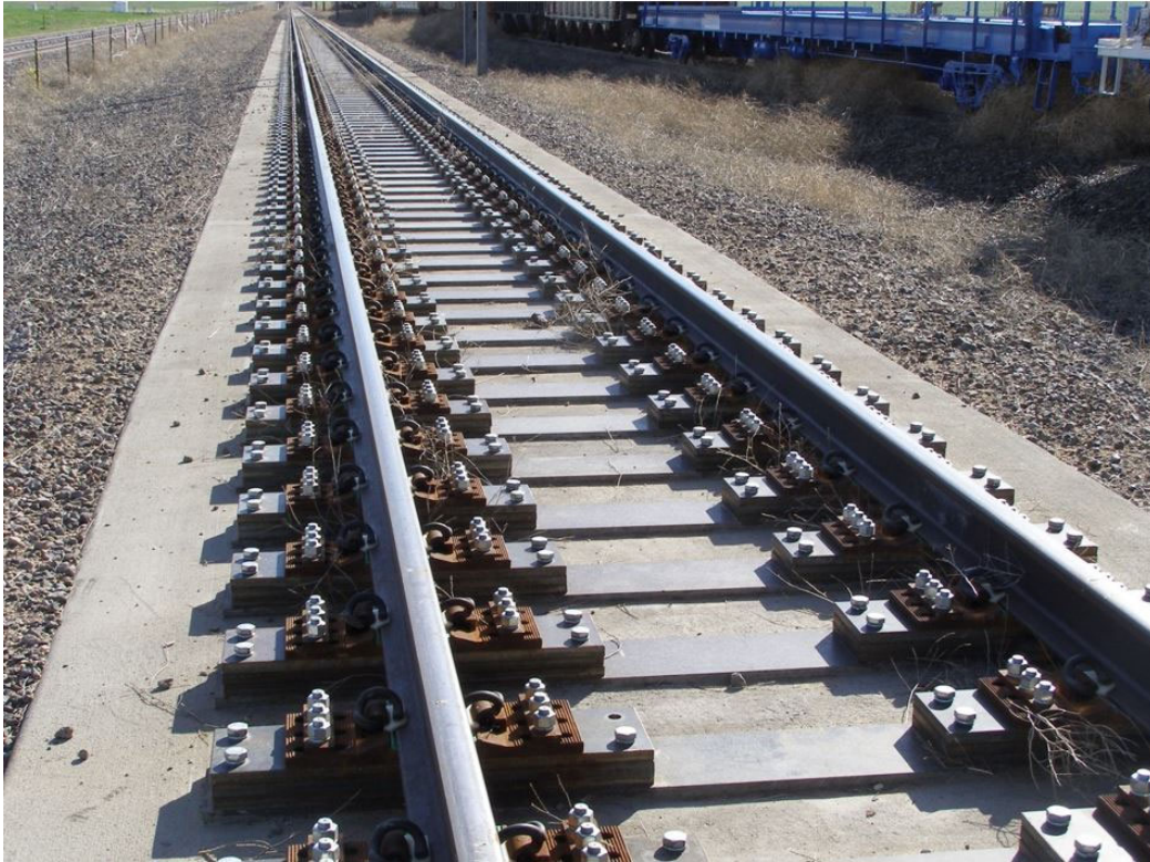
Figure 95. 500-foot Long HS-APS Test Track at the TTC
