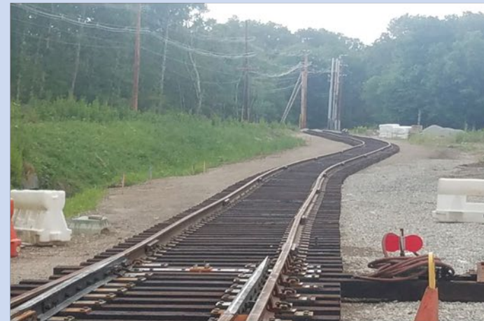
NER (Track Under Construction)
