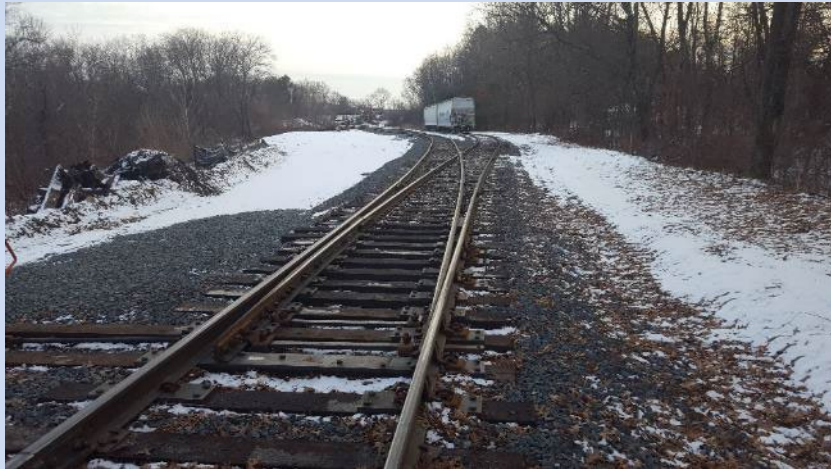
PVRR Easthampton Yard (New Siding)
