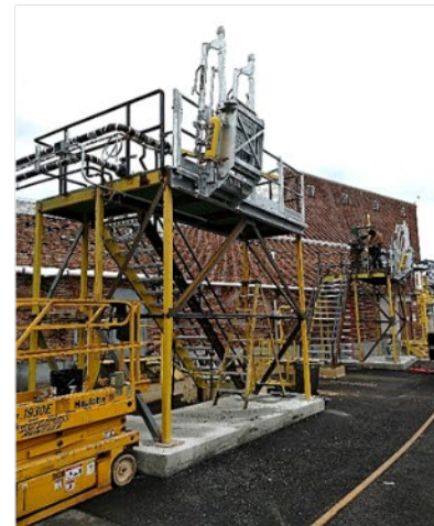
Boremco (Unloading Platform)
