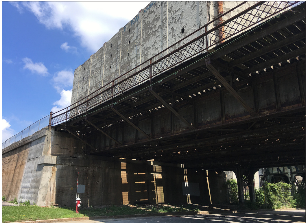
Centre Street Bridge South Elevation (View North) 1
