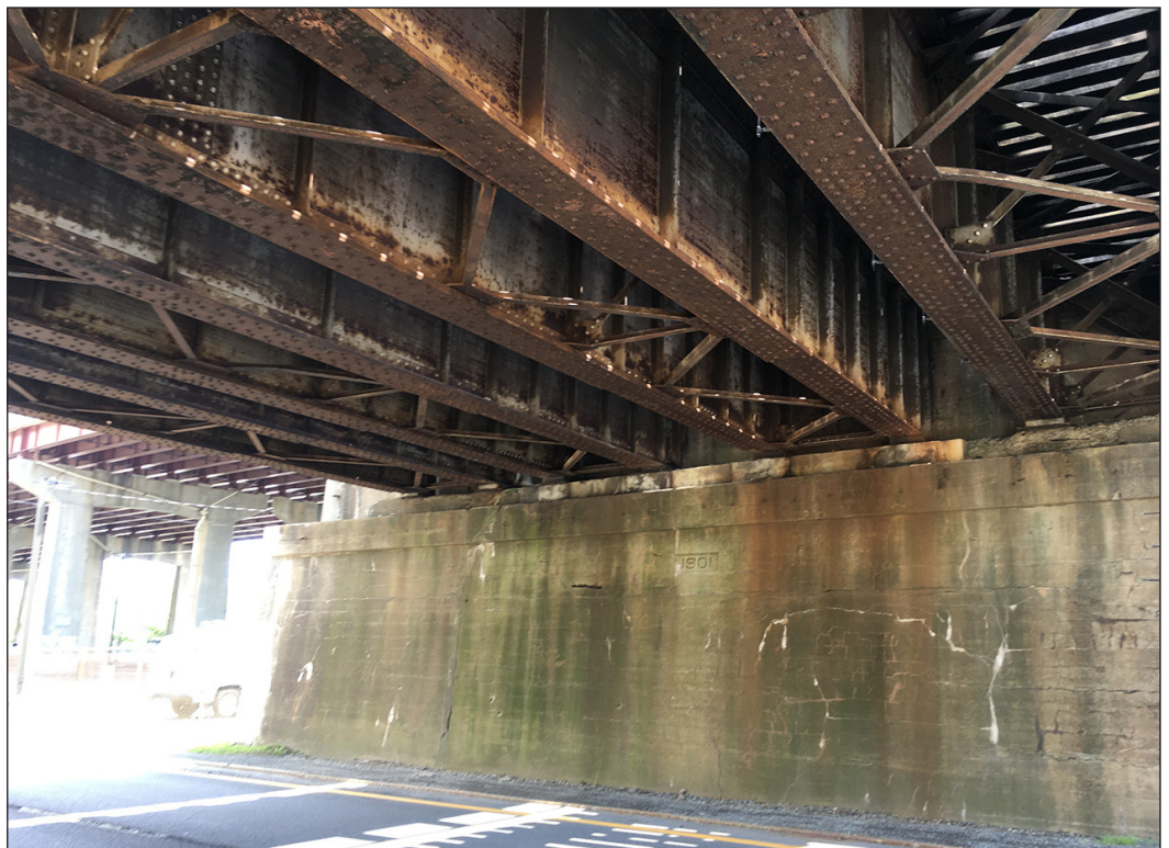
Water Street Bridge – East Abutment, Beam Seat, and Deck Girders 4
