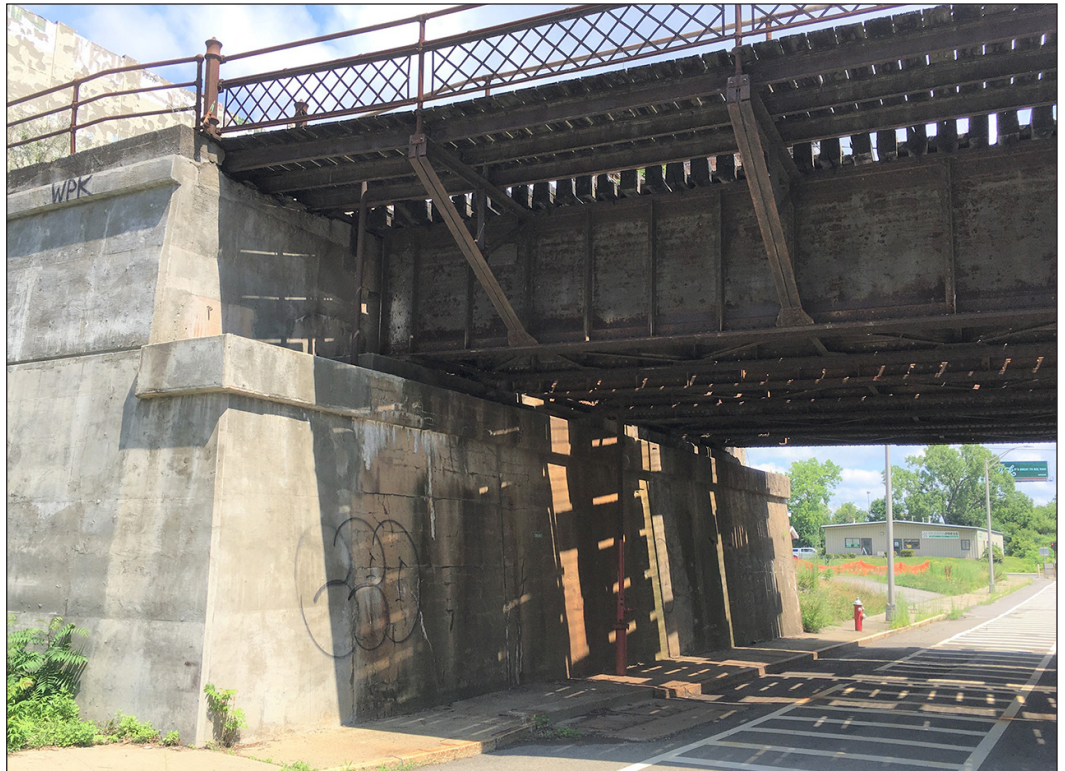
Water Street Bridge South Elevation (View North) 3
