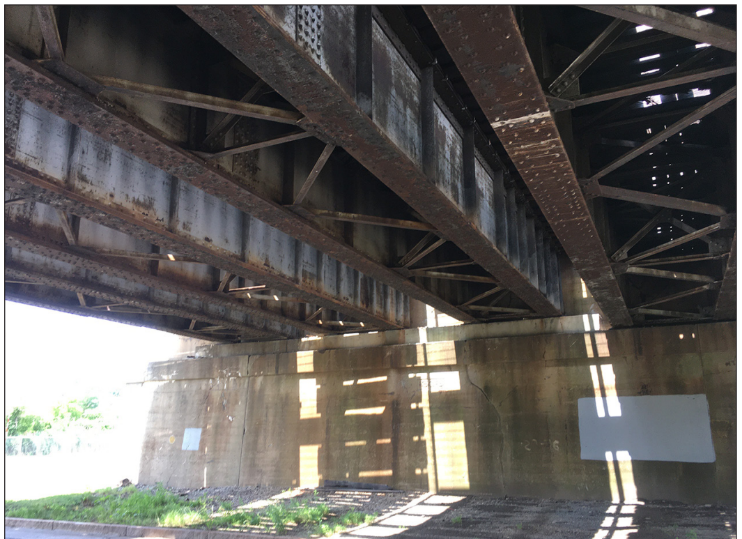
Centre Street Bridge West Abutment, Beam Seat, and Deck Girders 2
