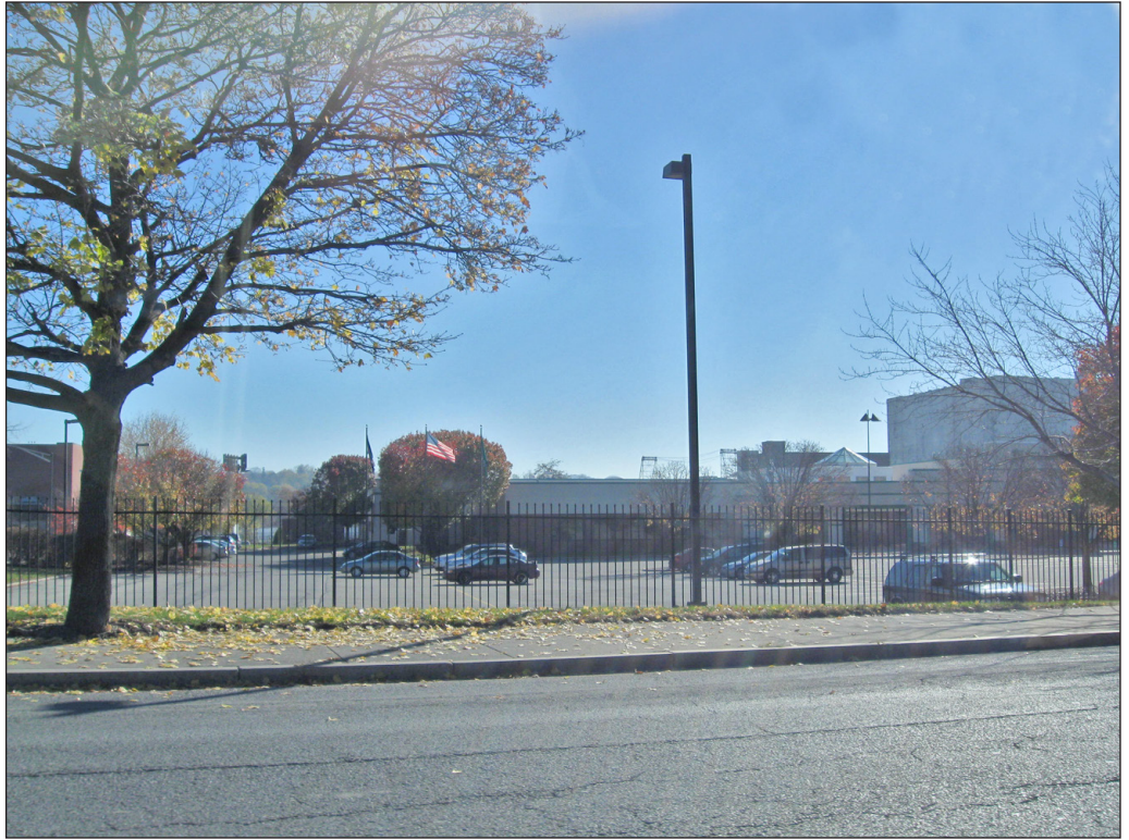
View looking east toward Livingston Avenue Bridge 7 from Broadway at North Lawrence Street
