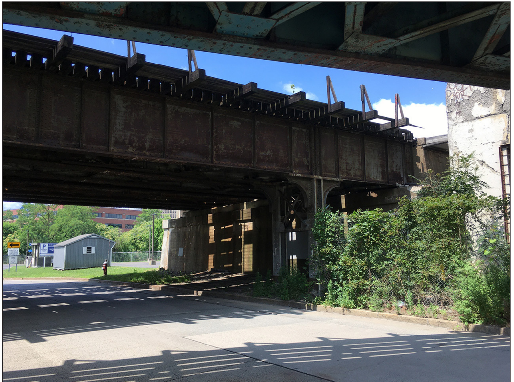
View south (north elevation), from beneath Centre Street Railroad Spur Bridge 6
