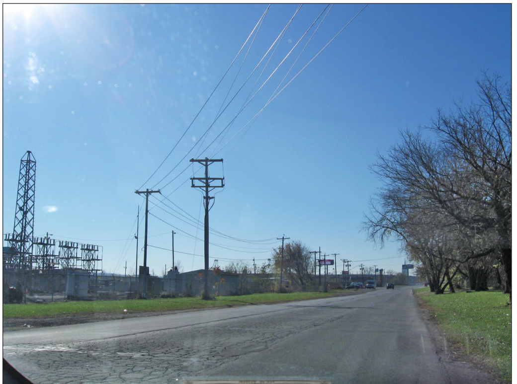
View looking south toward Livingston Avenue Bridge 6 from Erie Boulevard near Thatcher Street
