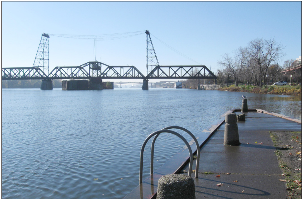
View looking south toward Livingston Avenue Bridge from Albany Boat Launch (NYSDOT owned property) 4
