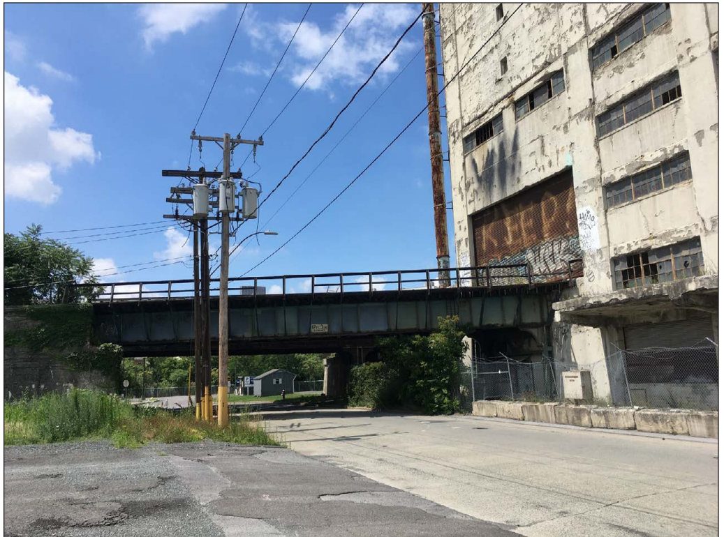
Centre Street Railroad Spur Bridge, view south on Centre Street 8
