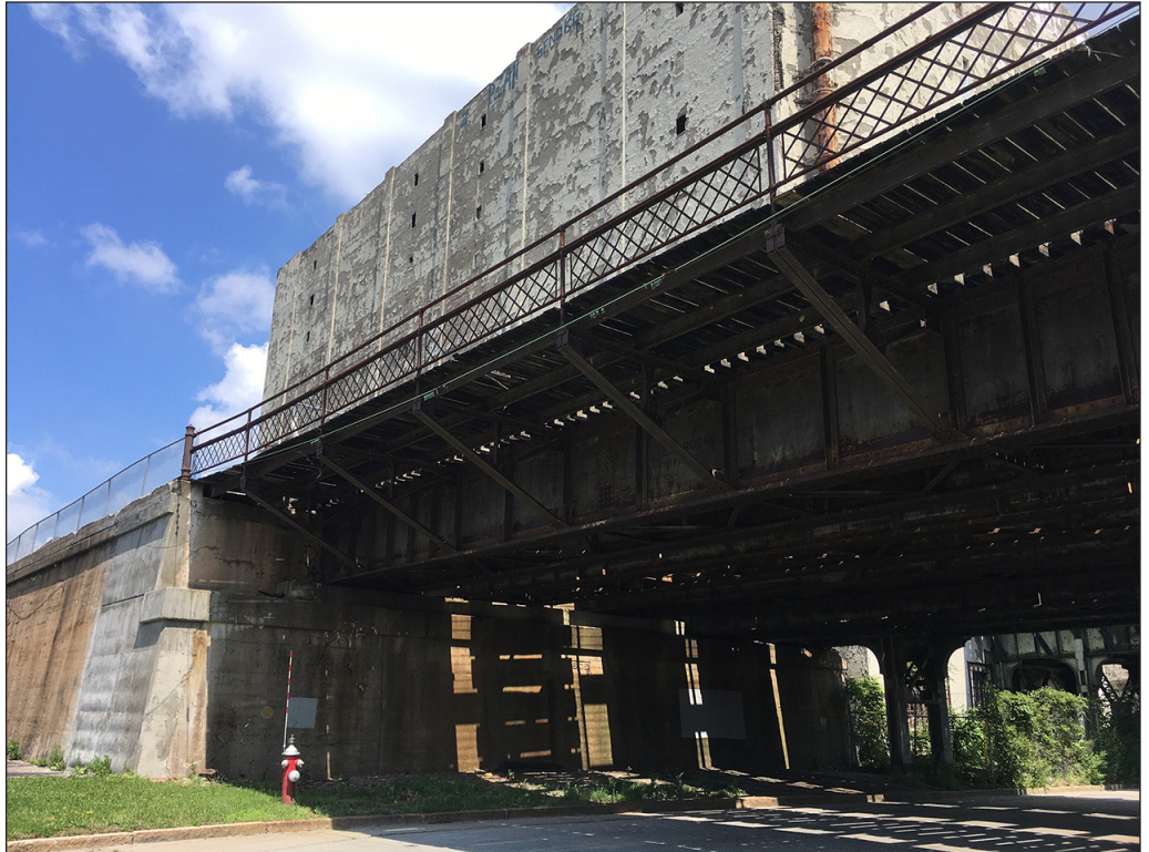
View north (south elevation), Central Warehouse in background 5
