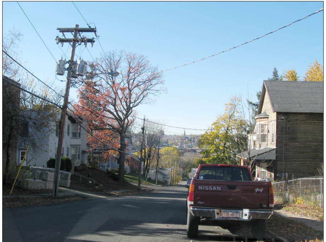
View looking west toward Livingston Avenue Bridge 10 from Macnaughton Avenue and Third Street
