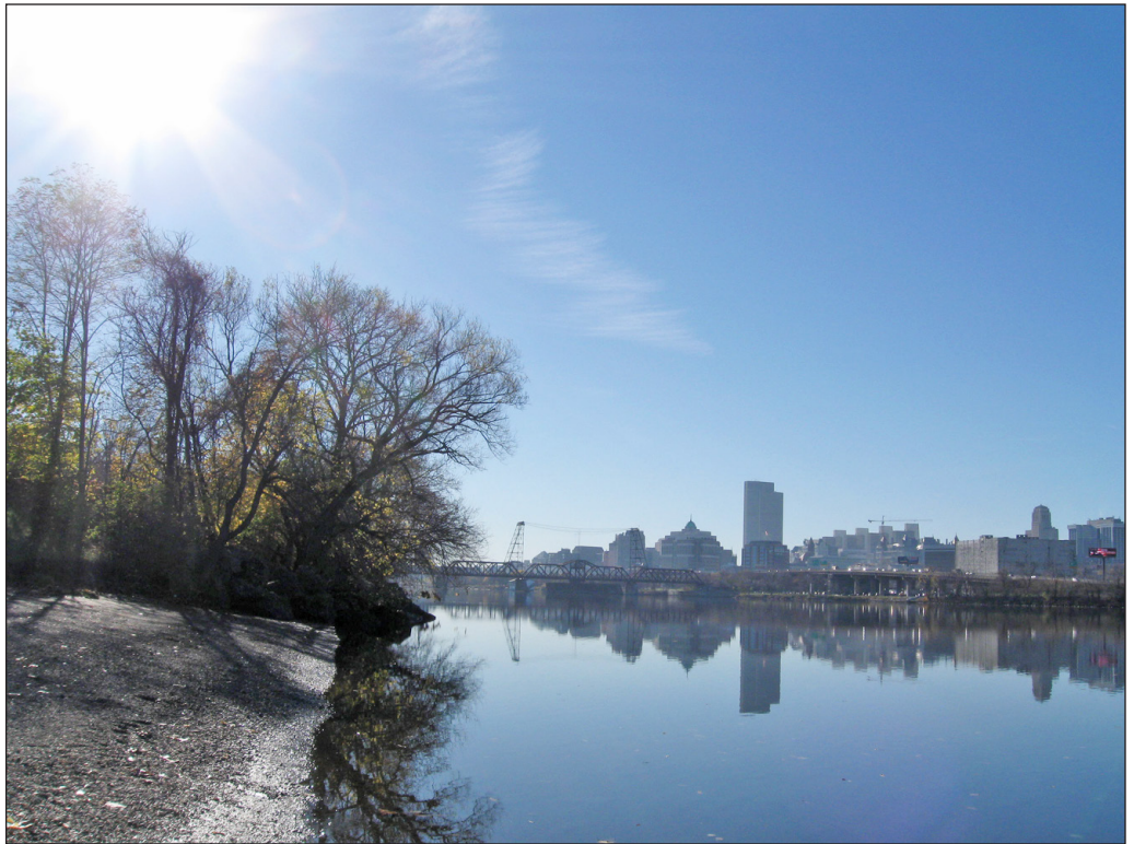
View looking south toward Livingston Avenue Bridge 8 from Rensselaer Boat Launch
