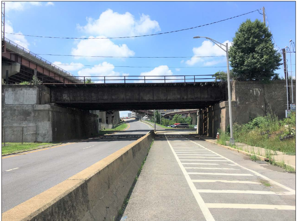
View south (north elevation) 4
