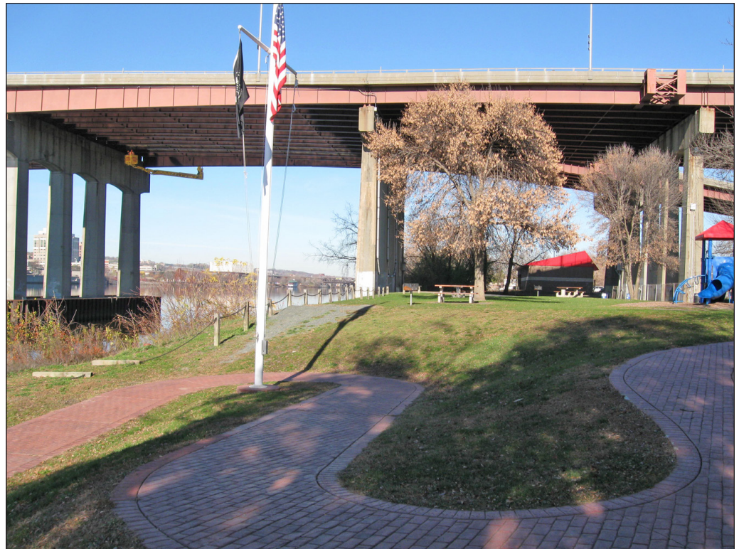
View looking north toward Livingston Avenue Bridge 12 from Riverfront Park (Rensselaer)
