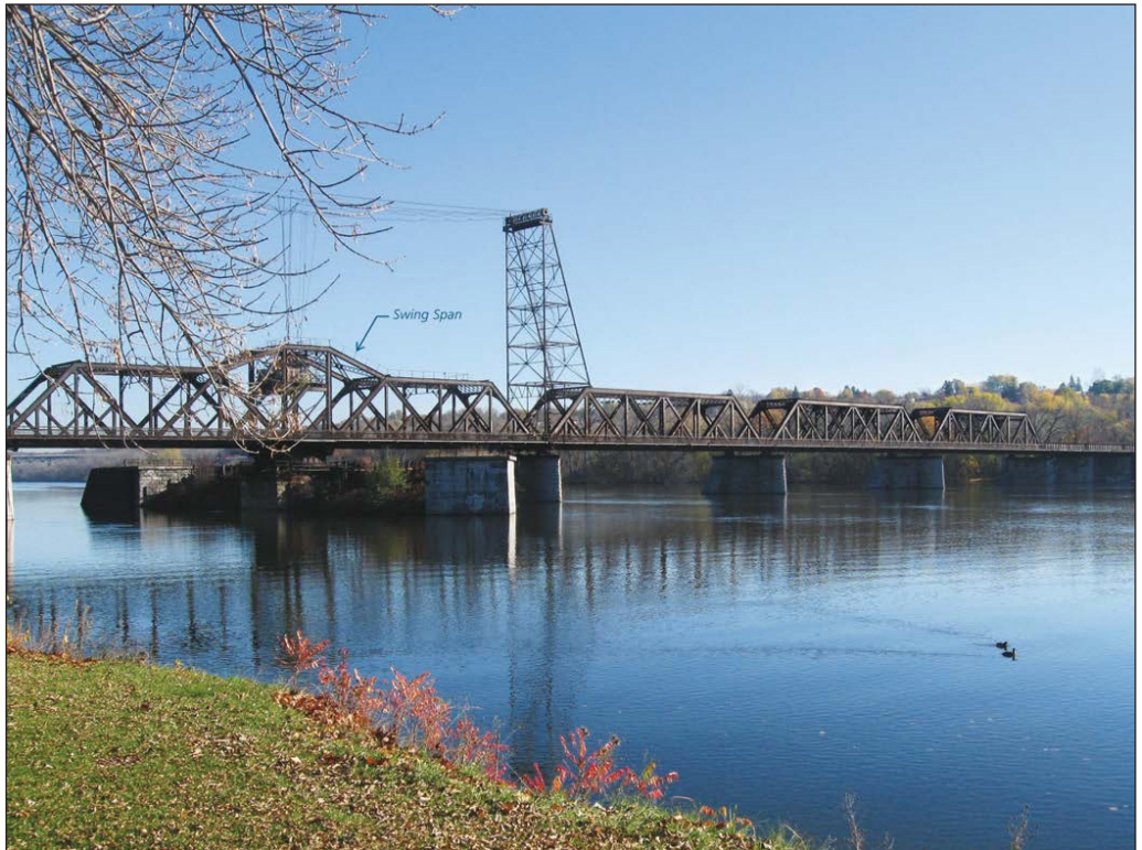
View looking east at the Livingston Avenue Bridge 1 from Corning Riverfront Park just south of the bridge
