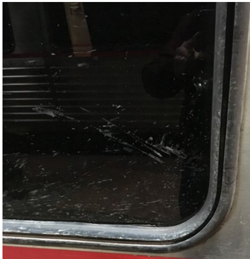
Figure 38. Exterior window with zip-strip removed
