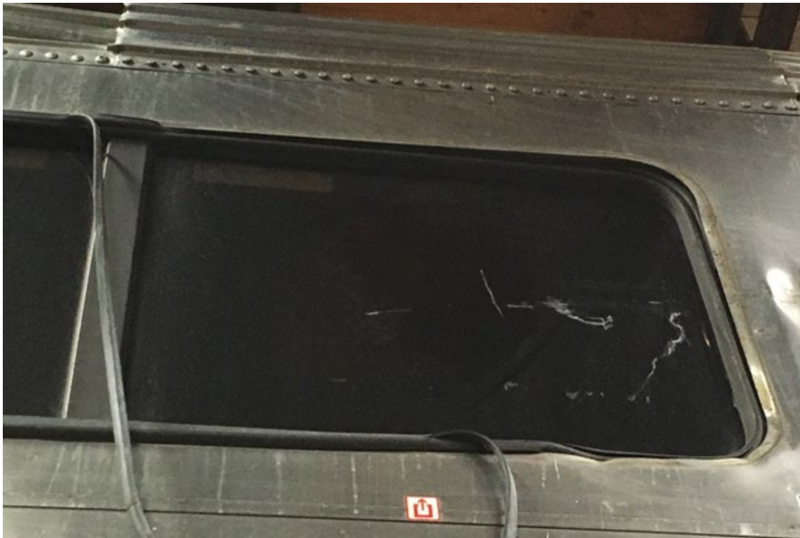
Figure 6. Zip-strip and gasket condition after accident, Cimarron, KS
