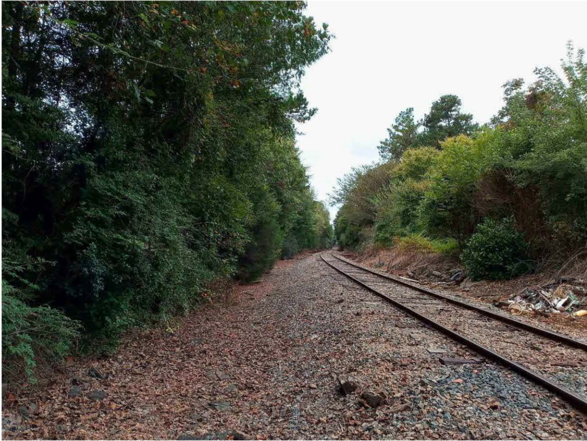
Photograph 3: View of Mint Hill Passing existing rail line and proposed rail corridor north of the existing line, western portion of the site, facing east.
