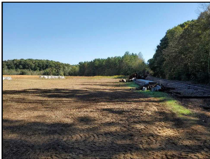
Figure 38: Cleared Portion of the Midland Siding Project Area, facing East
