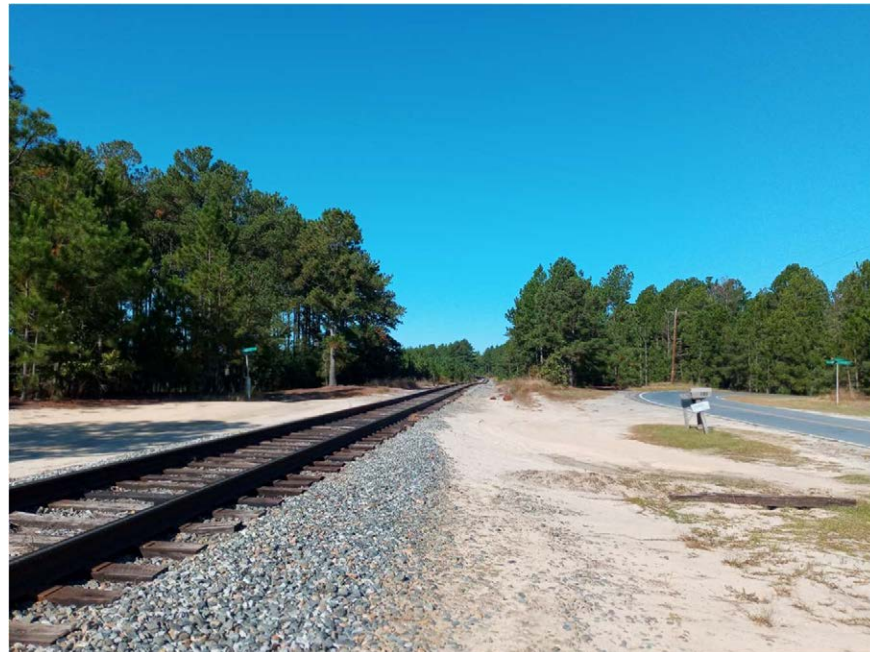
View of existing rail ROW, central portion, looking east.
