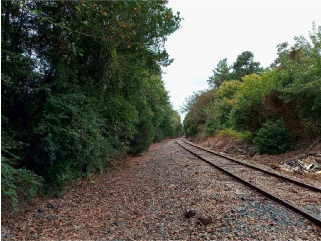
View of existing rail ROW, western portion of site, facing east.
