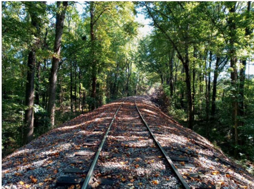
View of maintained rail ROW, northern portion of site, facing east.
