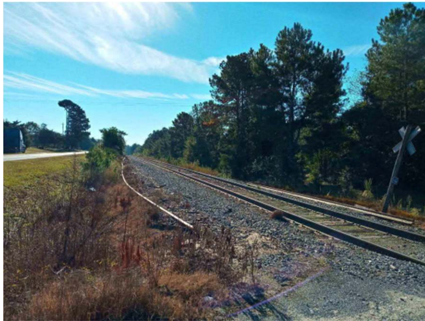
View of existing rail ROW, central portion of site, facing east.
