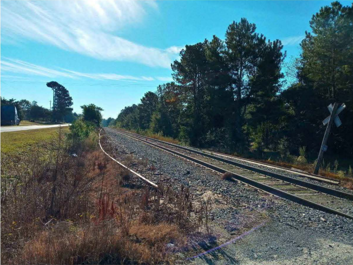
Photograph 5: View of Samarcond existing rail line and proposed rail corridor north of the existing line, central portion of the site, facing east.
