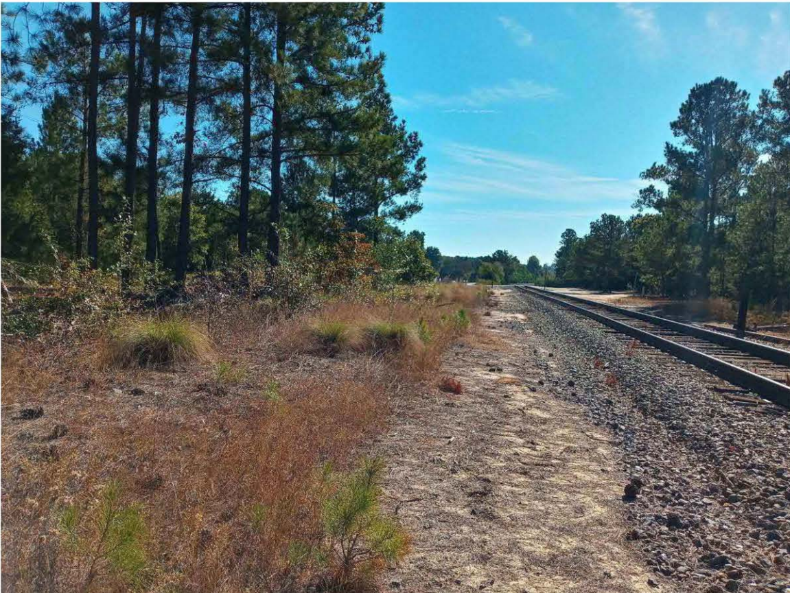
Photograph 6: View of Samarcond existing rail line and proposed rail corridor north of the existing line, eastern portion of the site, facing west.
