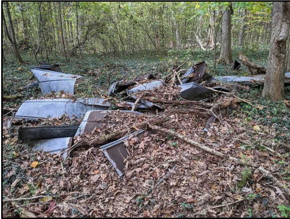
Figure 36: Metal Roofing at 31MK1173, facing North/Northwest
