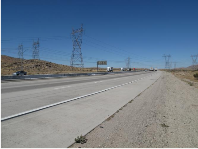
Segment 2, LADWP Boulder Lines 3, 2, and 1 (left to right), camera facing north, 8.5 miles northeast of Victorville, California and .5 miles northeast of Dale Evans Parkway at I-15
