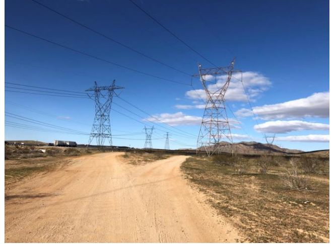
Access road (right) at Segment 2, camera facing northeast
