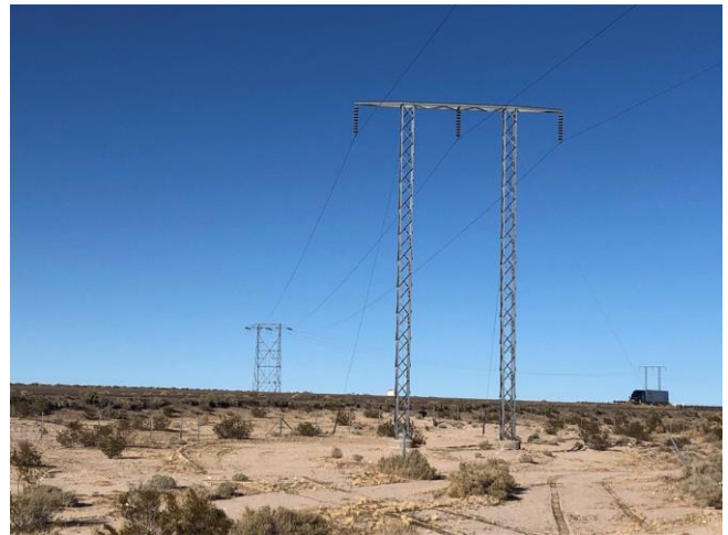
Segment 5, west end. Type H tower (foreground, south side), Type A dead-end tower (left, north side), Type H tower (background right, north side), camera facing north
