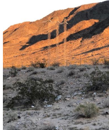
Segment 4, east end, south side. Type AP dead-end tower, camera facing east
