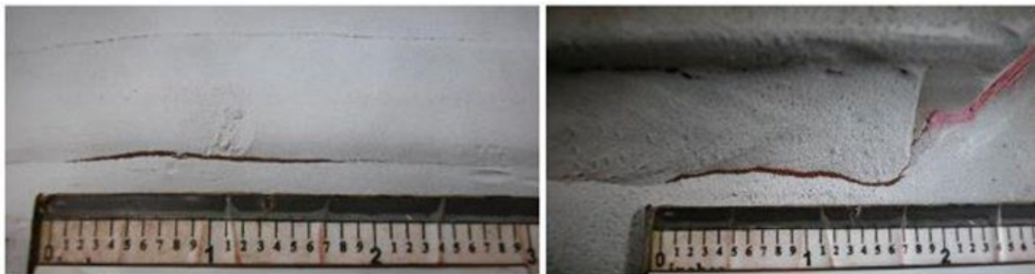
(a) (b) Figure 1. Contrast MT revealing toe cracking in welds of the DOT-111 master gauge test panel: (a) butt welds; (b) fillet welds
