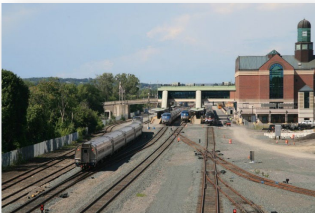
Exhibit 2-4 Interlocking CP 142 and New Fourth Station Track at Albany-Rensselaer, New York
