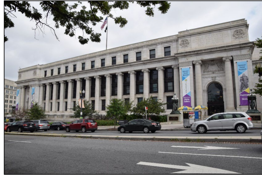
City Post Office south elevation
