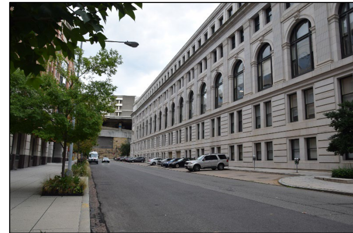
City Post Office north elevation, looking east
