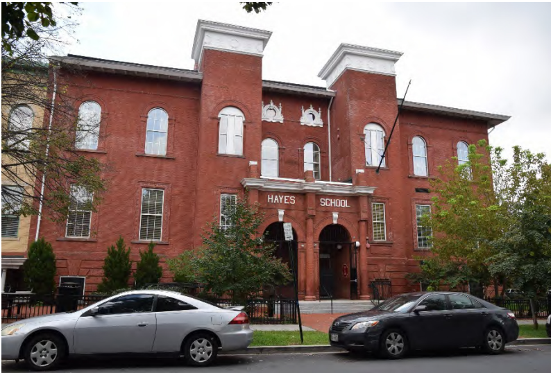
Hayes School, view looking east
