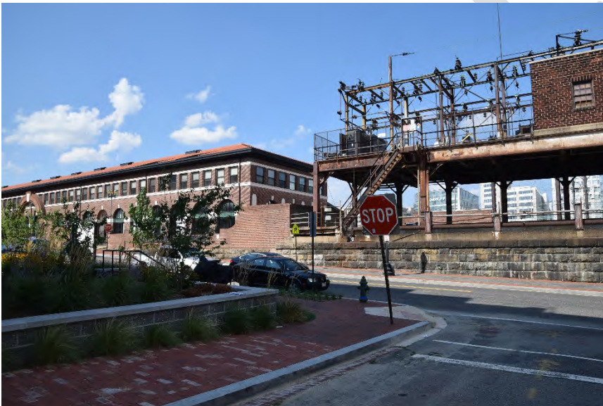
View from the west end of Parker Street within the Square 750 Rowhouse Development, view looking west towards Substation 25A the REA Building, both within the Project Area. Note that Substation 25A will be removed as part of another project, included in the No-Action Alternative.
