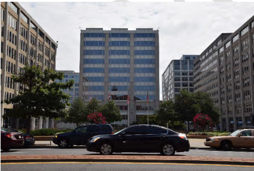
View from the east elevation of the church looking east towards the Project Area
