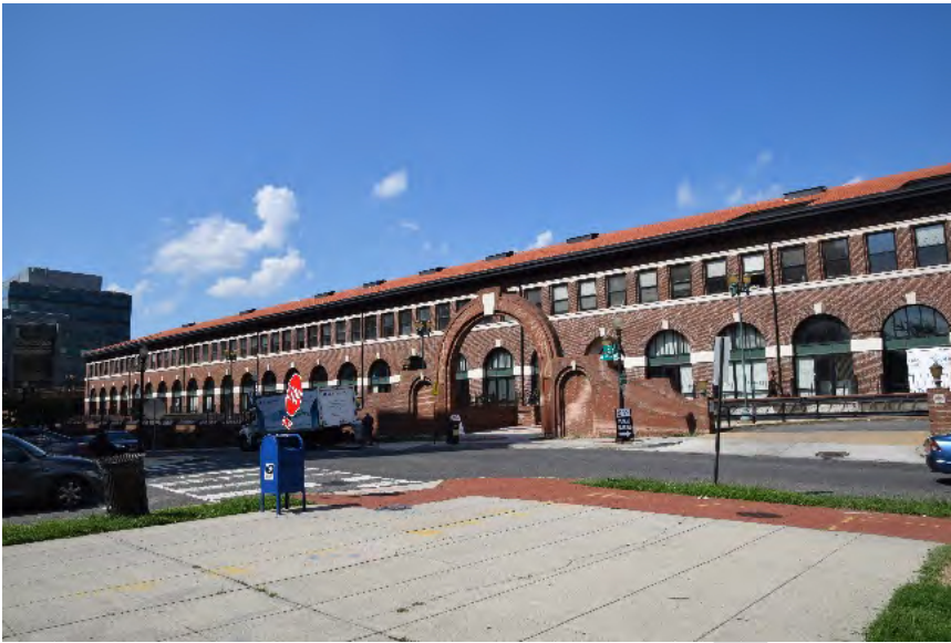
Railway Express Agency Building, view looking southwest
