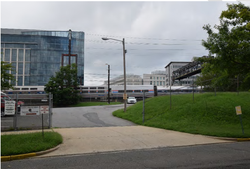
View from the west side of the building, looking west towards the Project Area. A signal bridge from the Terminal Rail Yard is visible on the right.
