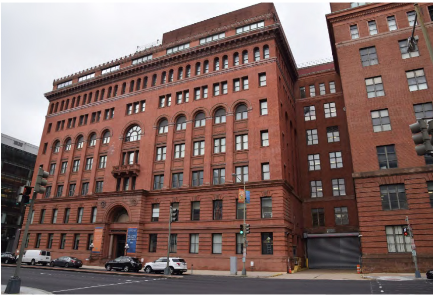
Government Printing Office, view looking west
