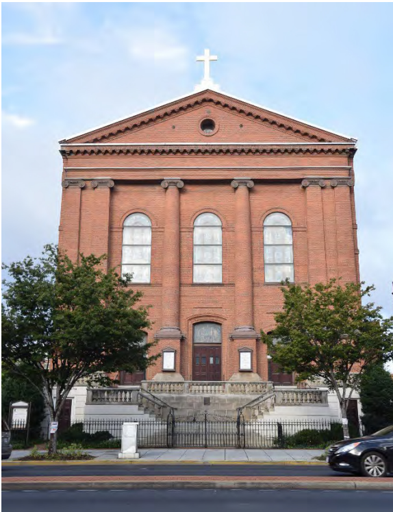
St. Aloysius Catholic Church, view looking west
