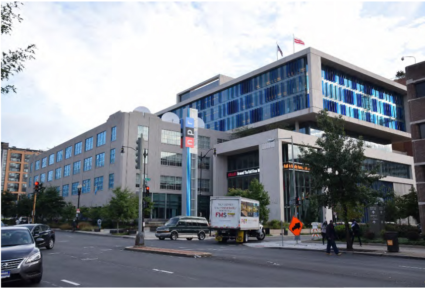
C&P Telephone Company Warehouse, view looking northeast from North Capitol and L Streets NW. The original building is on the left with an addition to the right.
