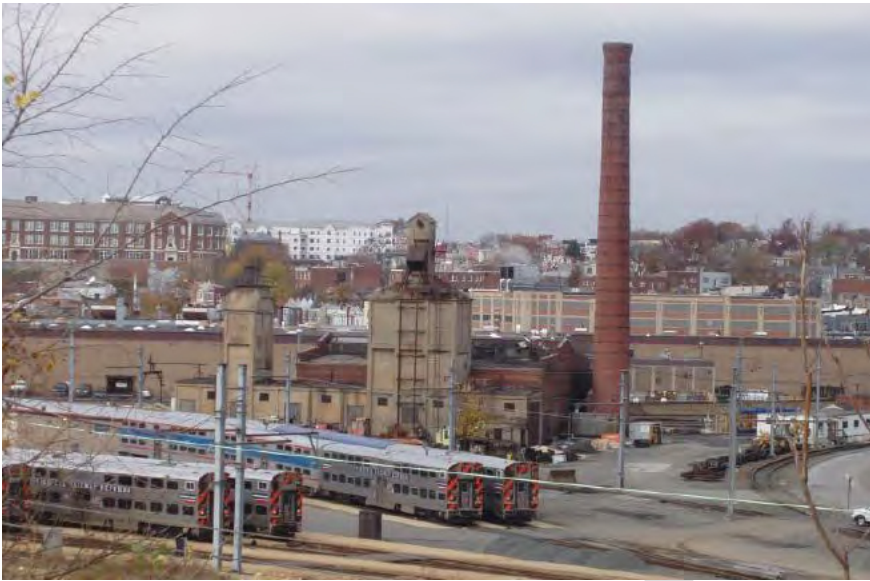
Eckington Power Plant, view looking west from New York Ave NE
