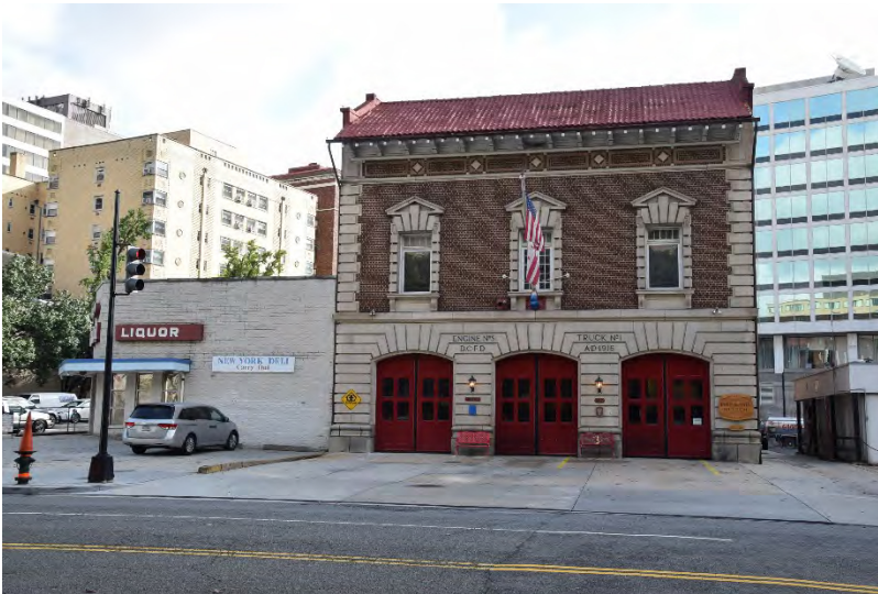
Engine Company No. 3 west elevation, view looking east from New Jersey Avenue. This property does not have a view towards the Project Area.
