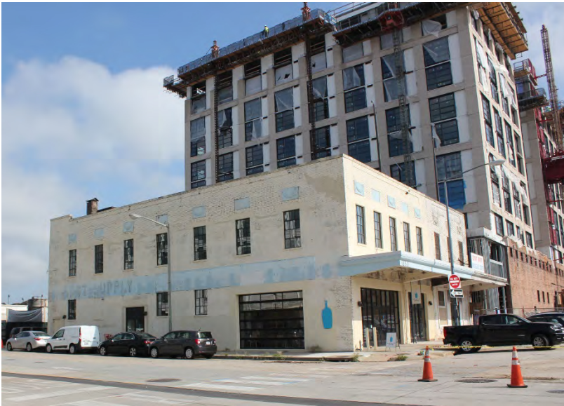
View of the Union Market Historic District looking northeast from the intersection of Morse Street NE and Fourth Street NE. The buildings are those within the APE.
