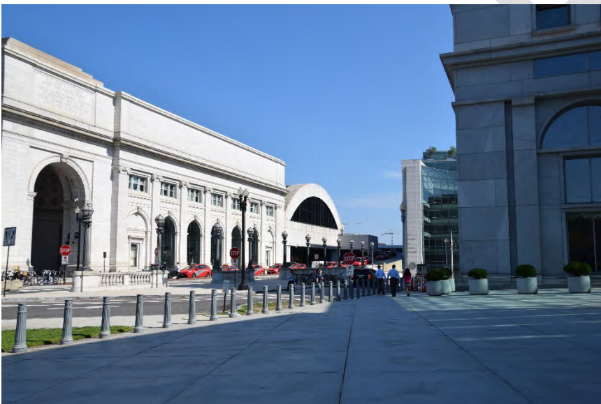
View from the west elevation of the property looking northeast towards the WUS headhouse and Project Area
