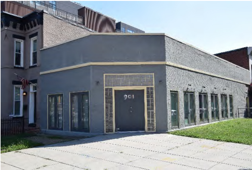
901 Second Street, view looking northeast
