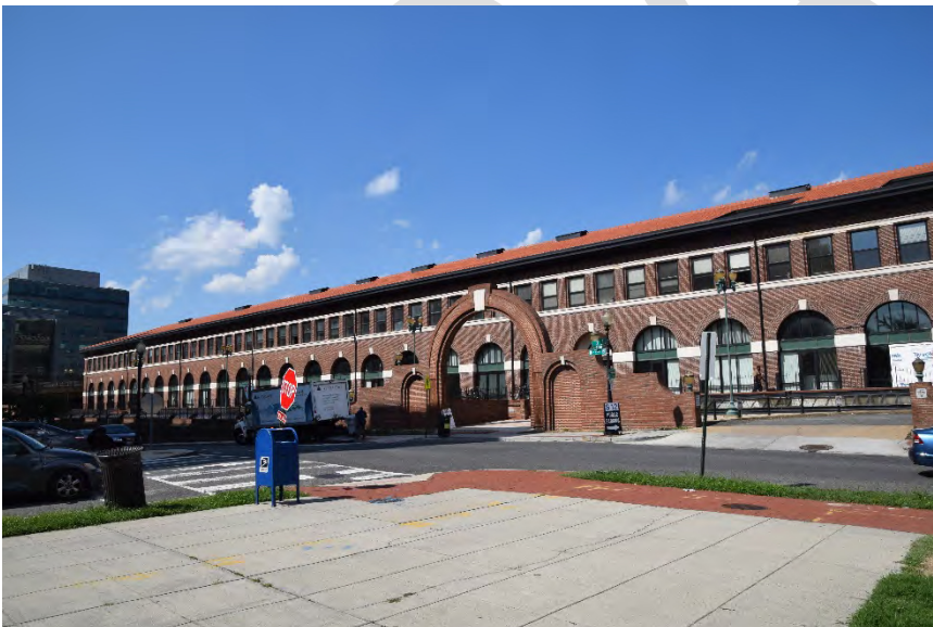
View from the corner of 901 Second Street, view looking west towards the REA Building and Project Area
