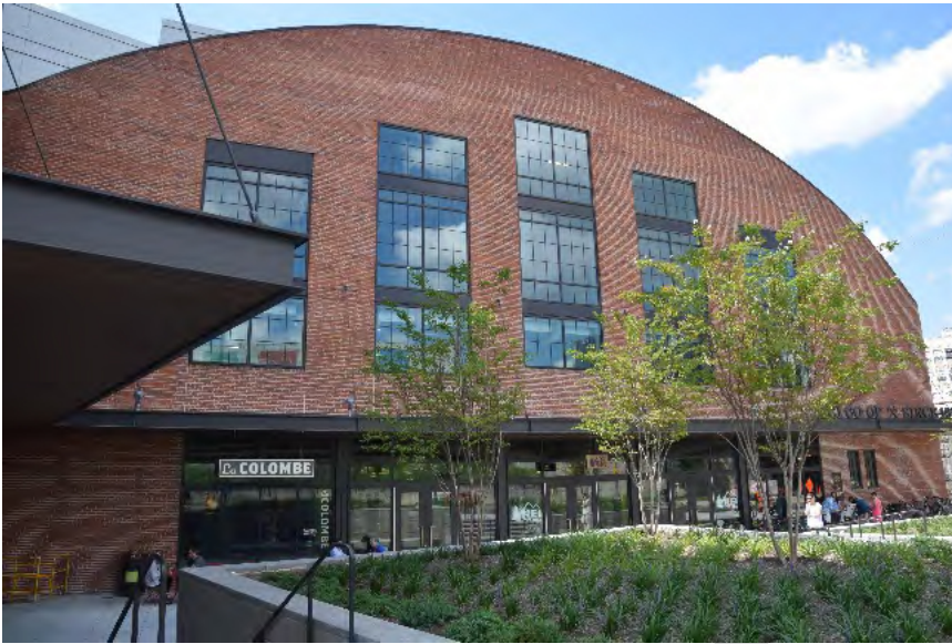
Uline Ice Company Plant and Arena Complex, view looking southwest
