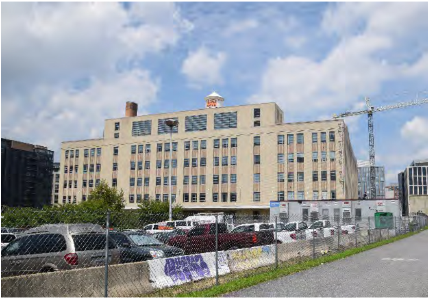
Woodward and Lothrop Service Warehouse, view looking north
