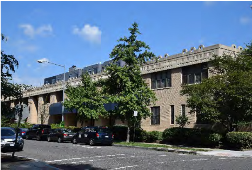
Topham's Luggage Factory (former), view looking northwest
