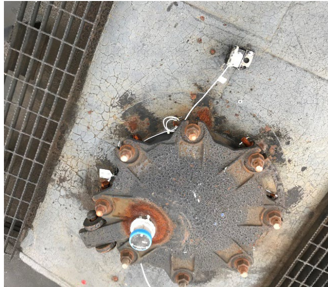
Figure 7. Triaxial Accelerometer Mounted on Top of the Carbody
